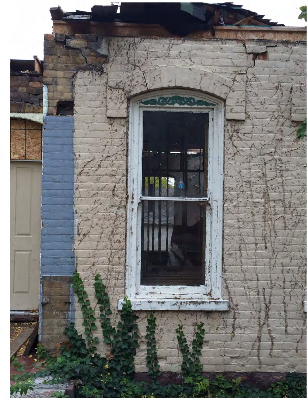
772 E. 2nd AVENUE CURRENT CONDITIONS NORTH WEST WINDOW 1A
