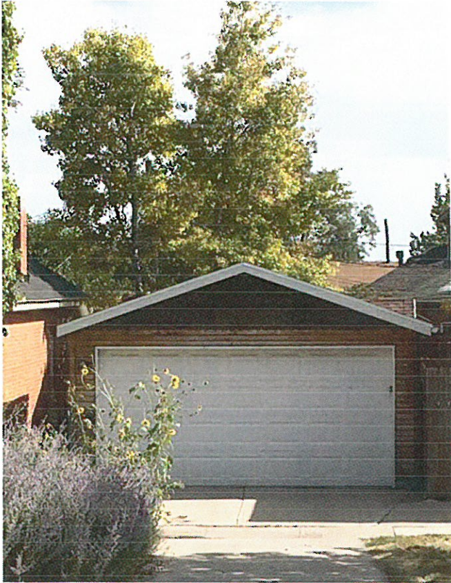
VISUAL AID - A: Image of neighboring existing garage located on 3rd Avenue. This view is looking South from 3rd Avenue. This image shows the current view and building corridors between the adjacent structures.
