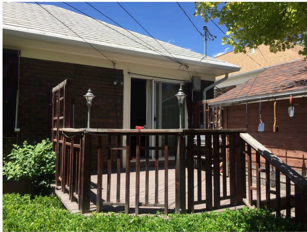
3 LOOKING WEST AT REAR OF (E) RESIDENCE AND DECK A4.0
