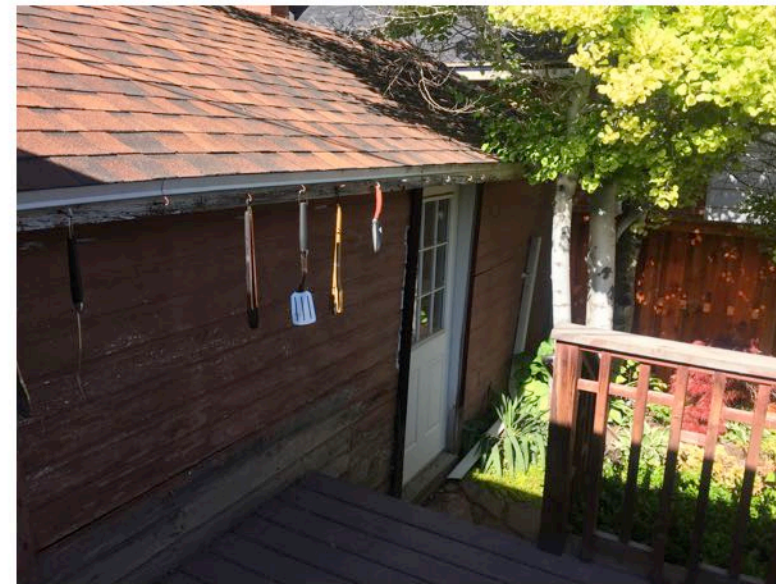
2 LOOKING EAST AT REAR YARD AND (E) GARAGE A4.0
