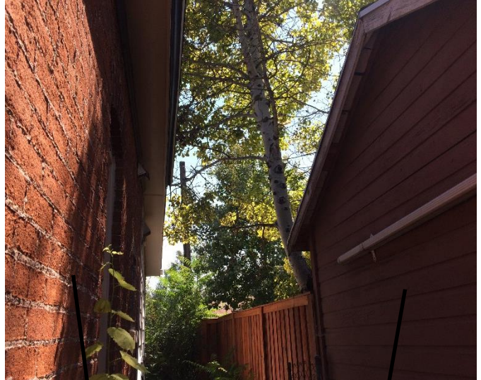
Primary structure closer than 10 FT on adjacent lot to the east
