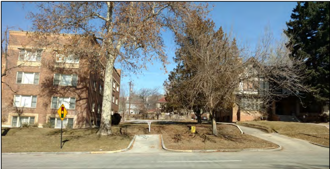
Street View of Subject Property from South Temple Street
