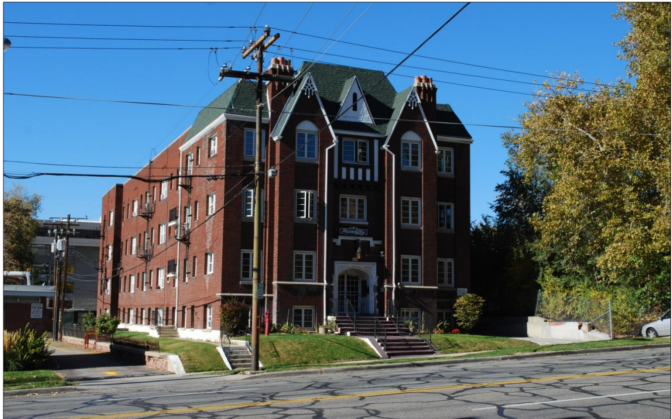
PICCADILLY APARTMENTS, 24 SOUTH 500 EAST
