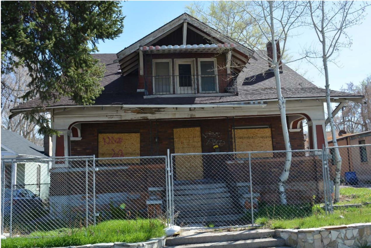
View from sidewalk along 300 West
