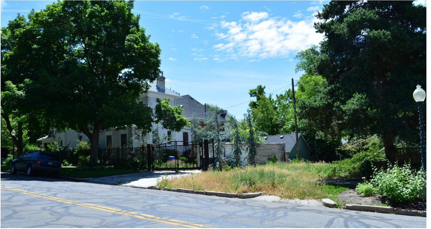
View from 2 nd Avenue of subject property and adjacent structures to the east.
