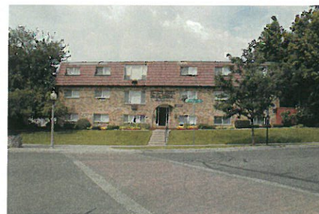
155 N Canyon Road** D
