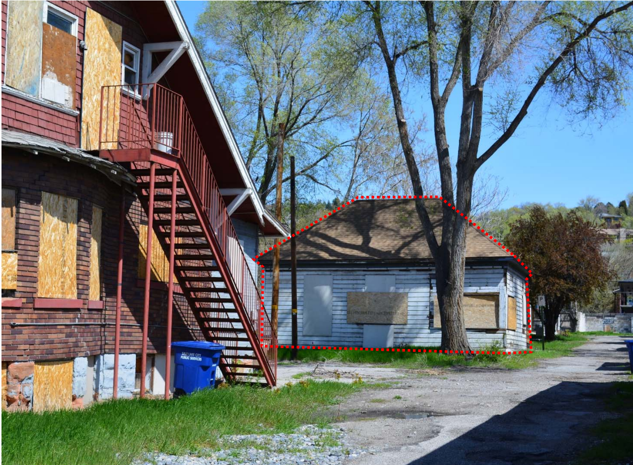
View from sidewalk along 300 West, Subject Structure highlighted
