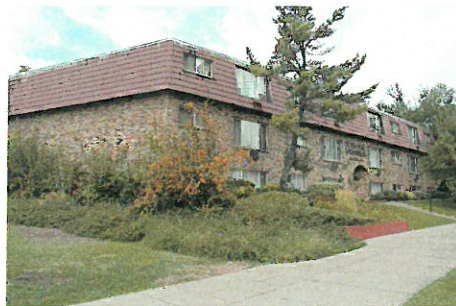
135 N Canyon Road** D
