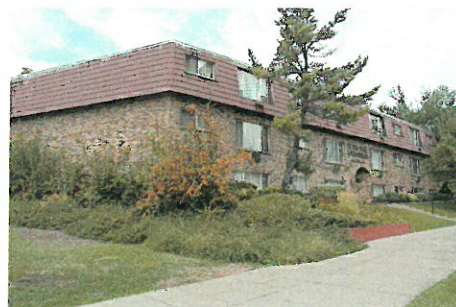
135 N Canyon Road** D
