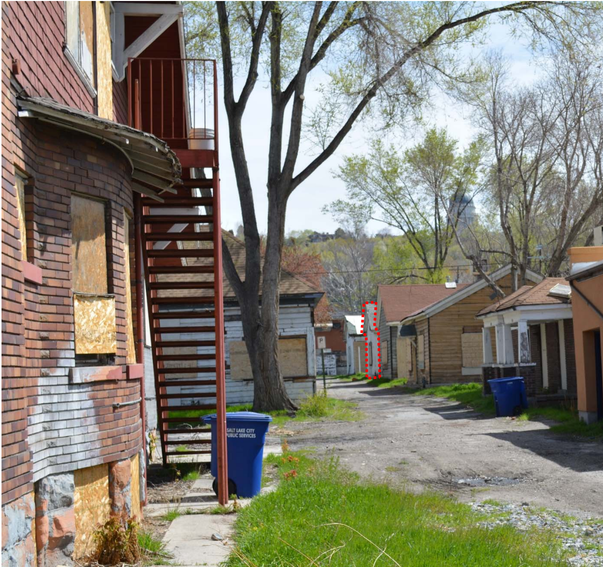
View from sidewalk along 300 West, Subject Structure highlighted
