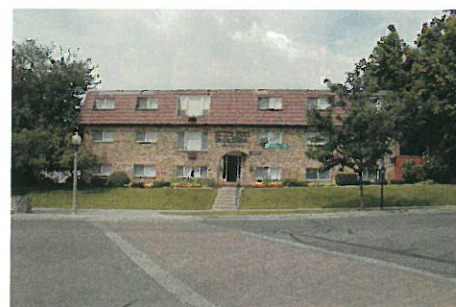
155 N Canyon Road** D
