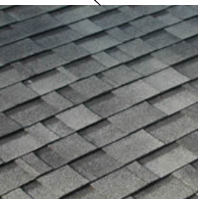
Asphalt Shingles - Garage Roof
