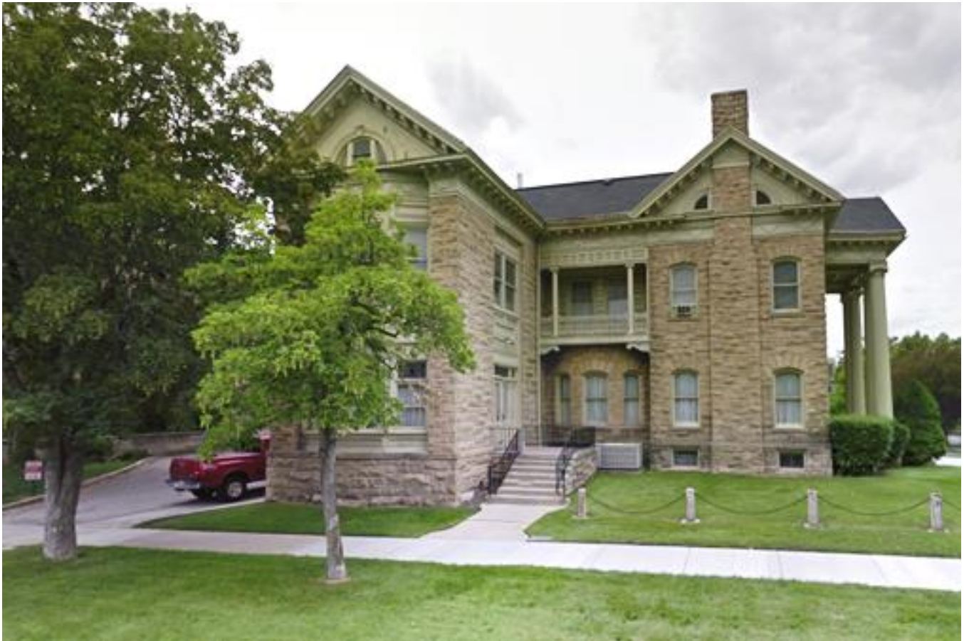
Current view of the East Porch
