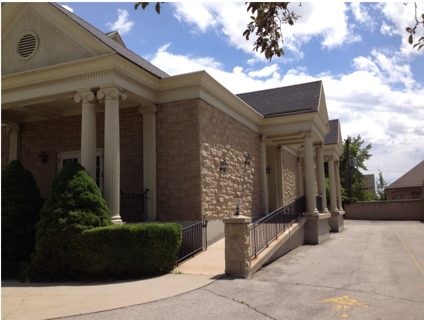
West façade, 1972 addition to be removed.
