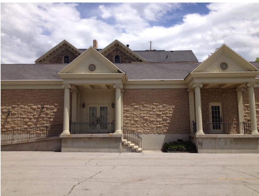
West façade, 1972 addition to be removed.
