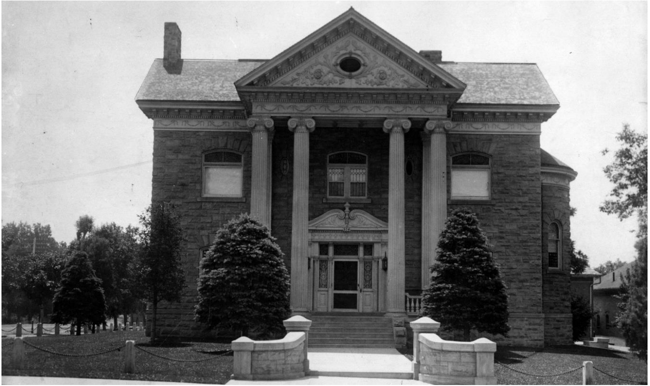
North Elevation, before 1937
