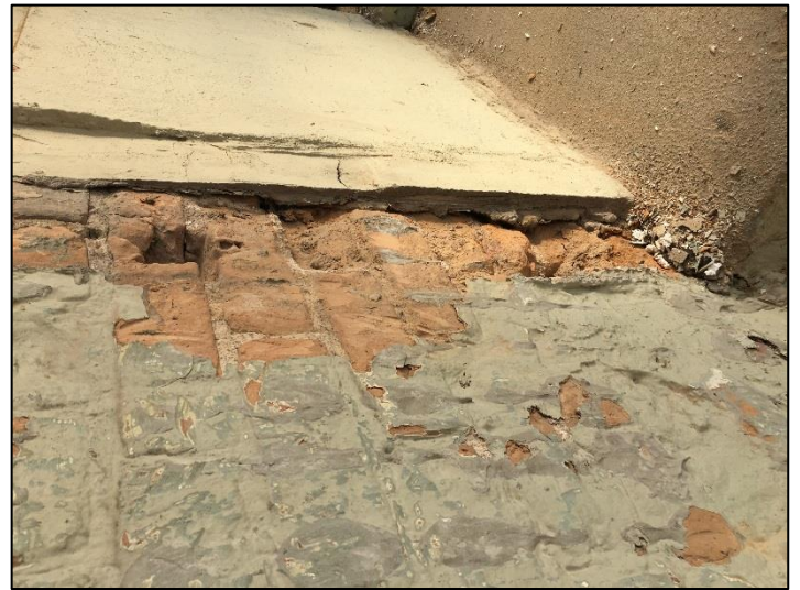
Illustration of the Brick Damage
