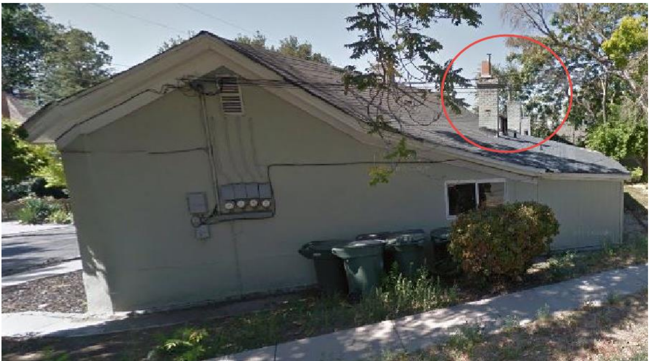
Photo Illustrating the Previous Chimneys
