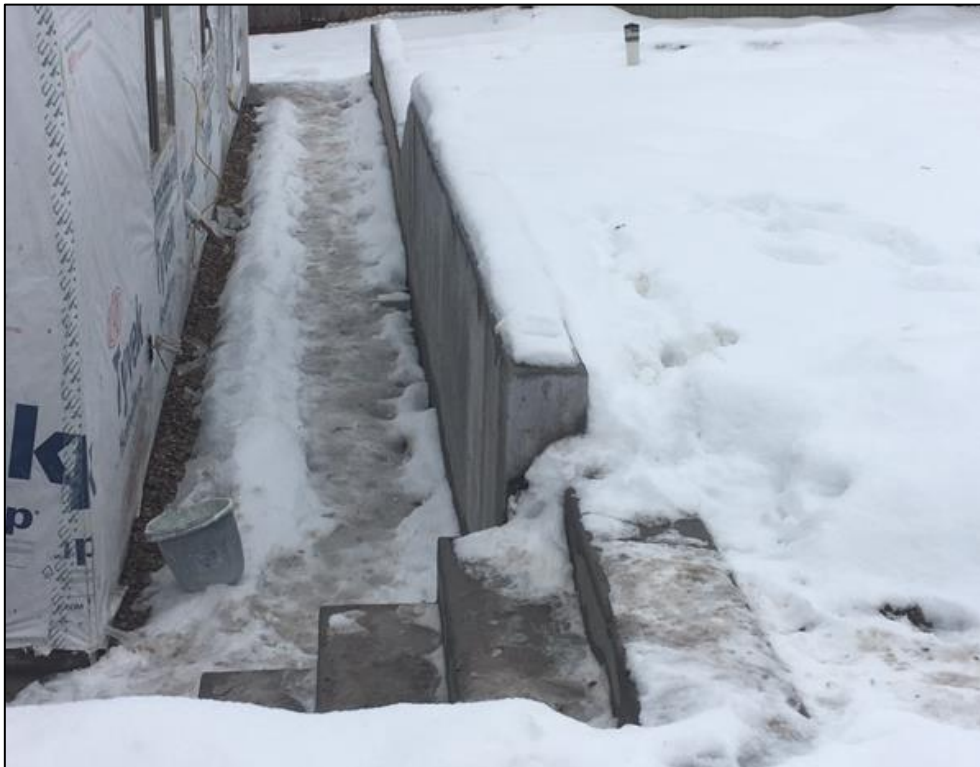
Retaining Wall and Stairs
