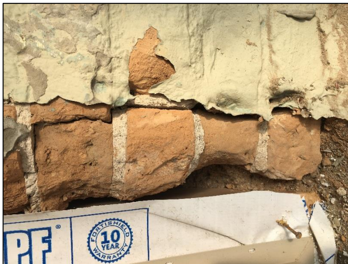
Illustration of the Brick Damage
