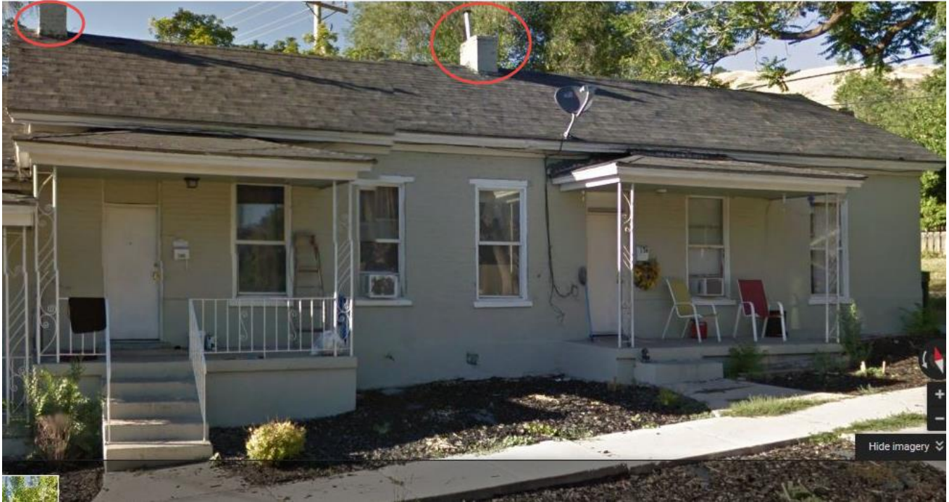
Photo Illustrating the Previous Chimneys
