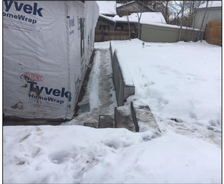
Constructed Retaining Wall
