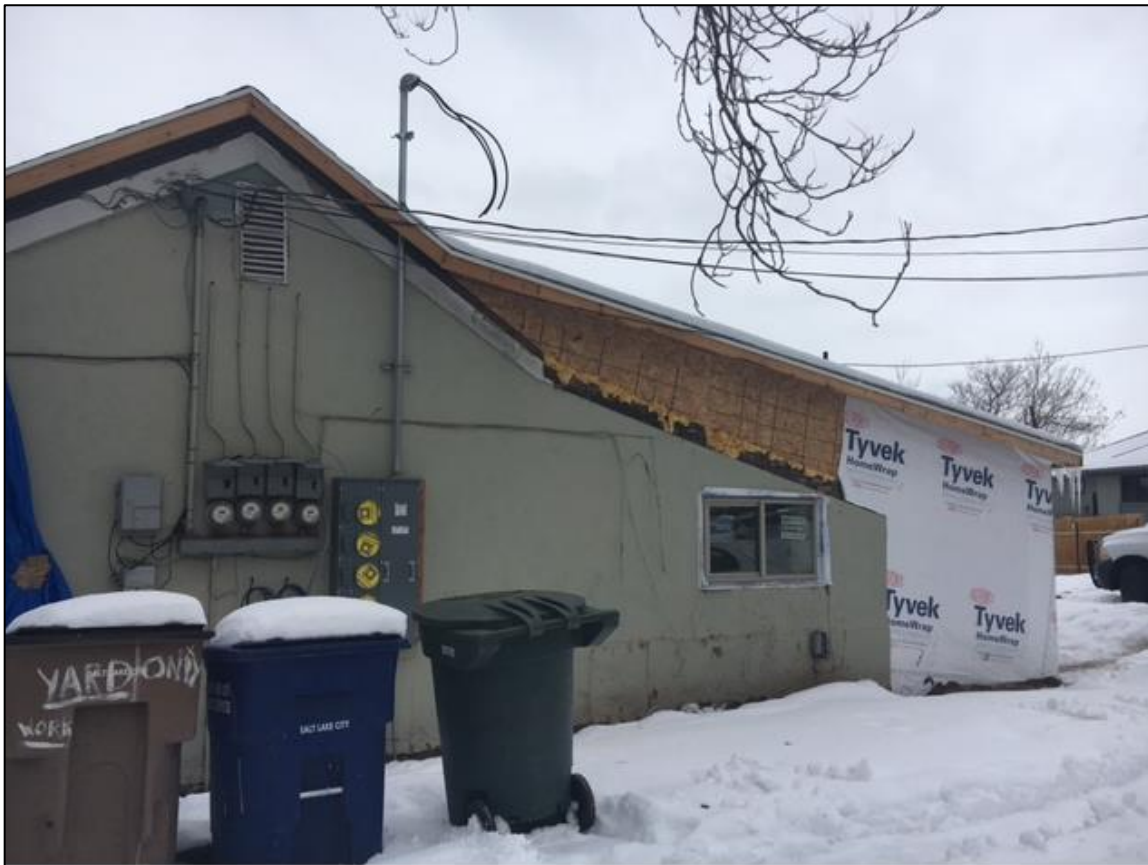
East Elevation Roofline Constructed
