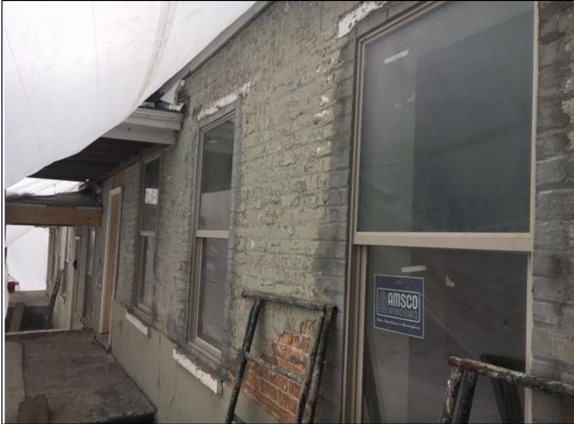
Vinyl Single-Hung Windows Installed
