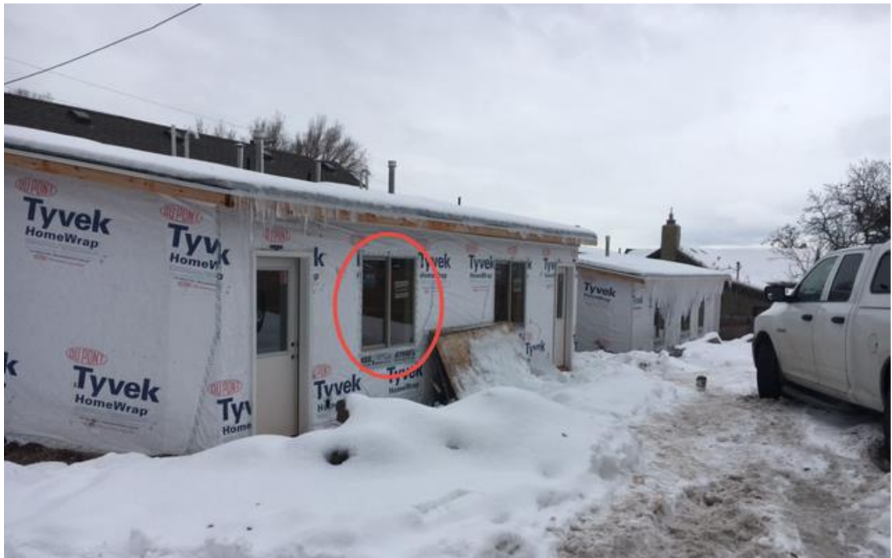
Illustration of the Installed Vinyl Sliding Windows
