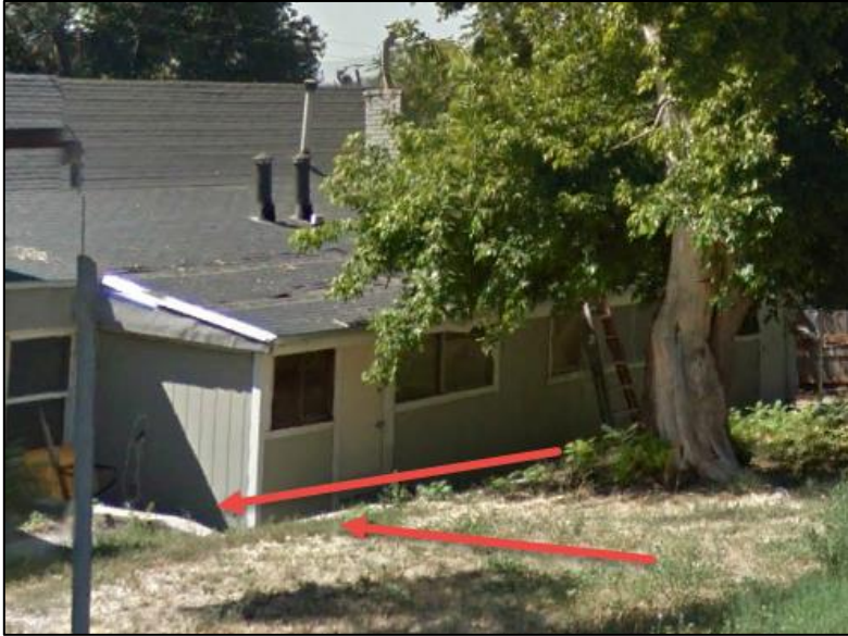
Previous Retaining Wall
