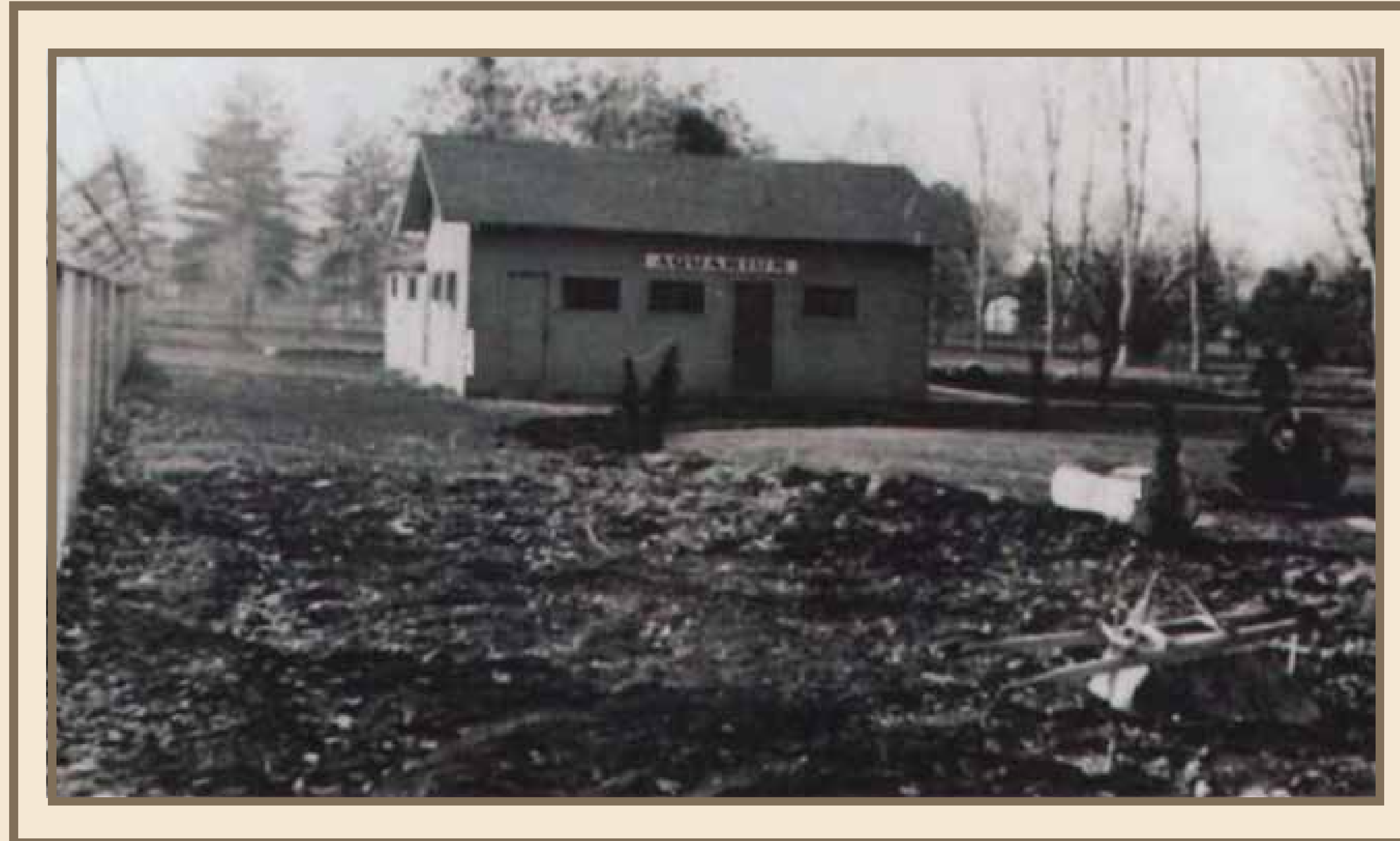
A picture from 1938-39 shows the structure from the East with an "Aquarium" sign.
