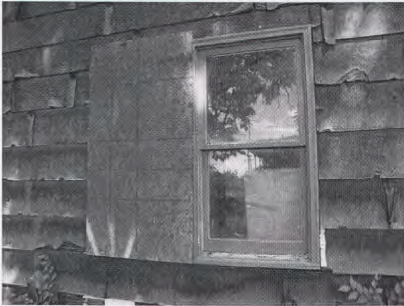
West side of home. North window has been expanded and replaced.
