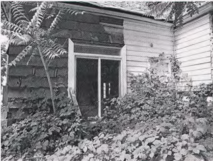
A vinyl slider has been installed. New framing evident.
