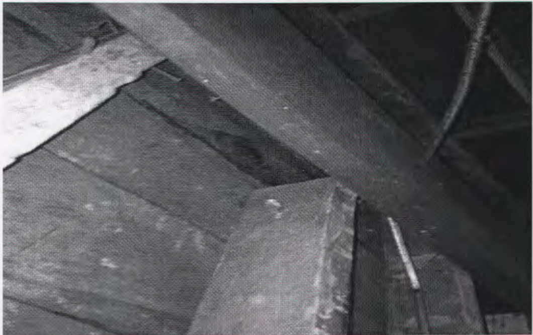
Photo 5: Cut wall stud
