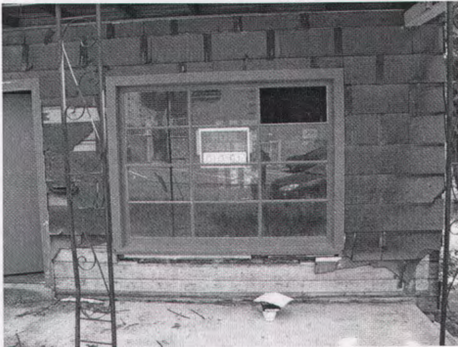
North Porch Window
