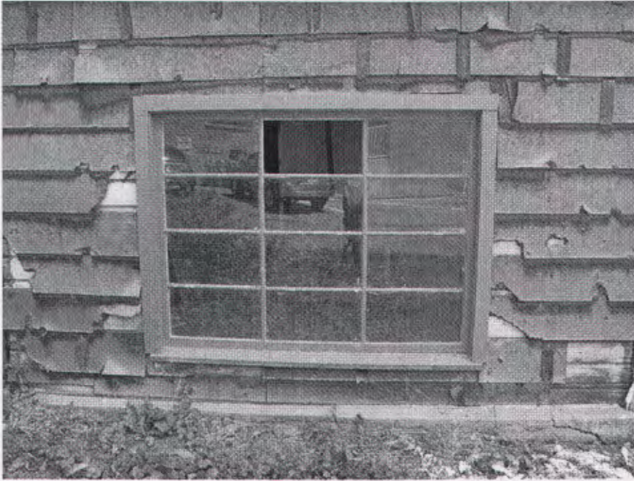
North front of home window.
