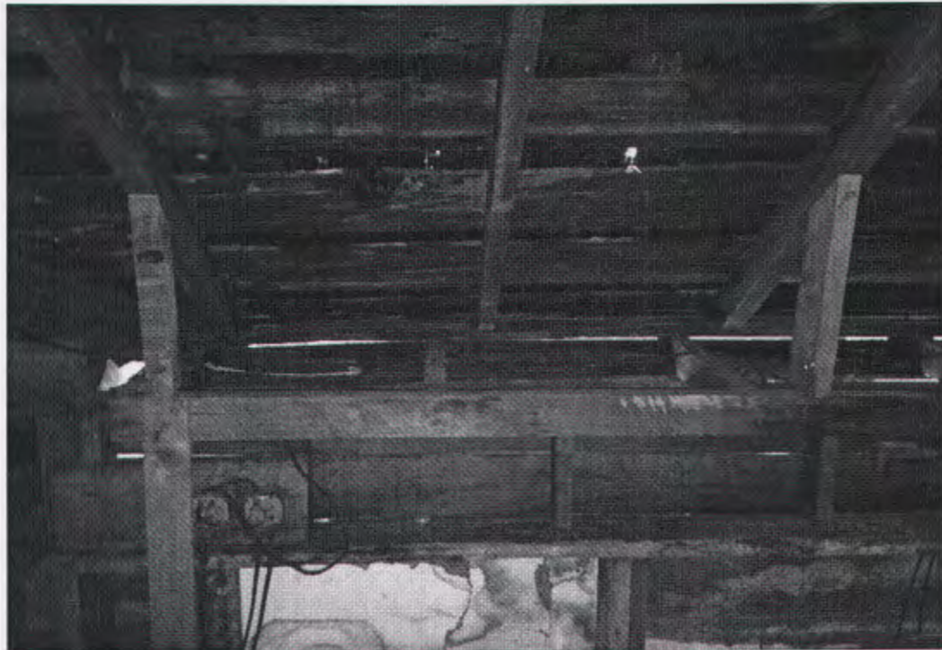
Photo 4: Cut rafter ties
