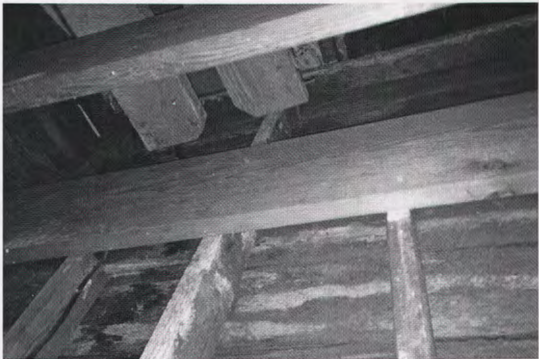
Photo 6: Cut wall studs
