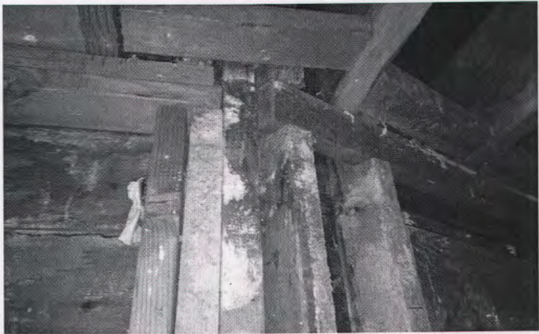
Photo 10: Cut wall studs
