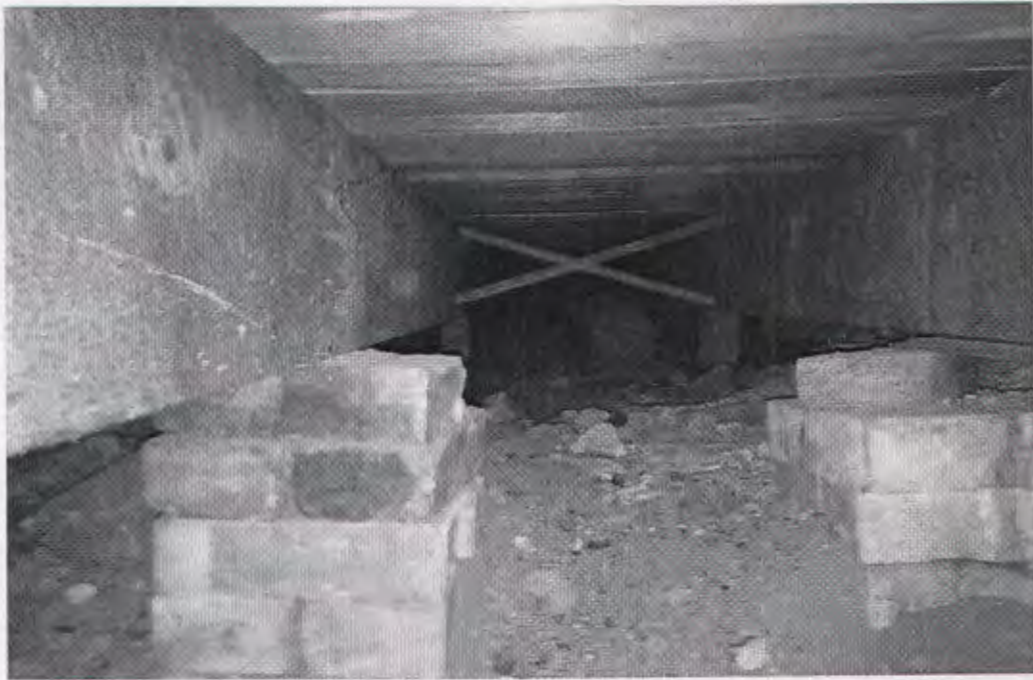
Photo 7: Brick pier footings
