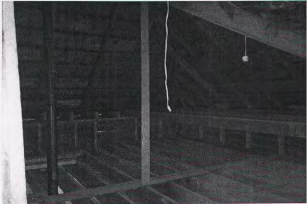
Photo 3: Second floor framing
