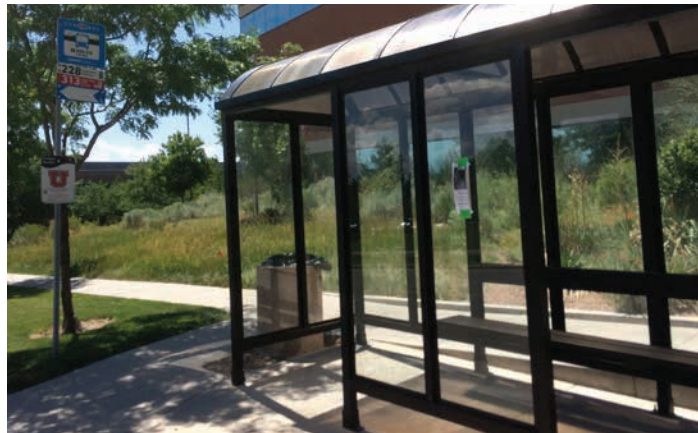
Enhanced bus stops, such as this bus shelter in Research Park, provide comfort and shelter for riders
