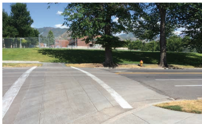
Raised crossings, such as this one near Uintah Elementary, are one traffic calming element that can make routes to school safer.
