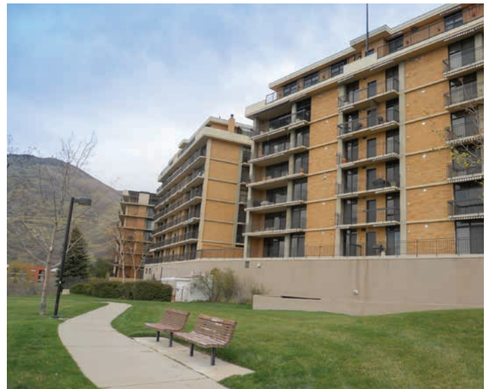
The majority of the East Bench community is typified by low-scale single-family residential development. The northeast corner of the East Bench neighborhood is unique in having a number of taller apartment and condo buildings.
