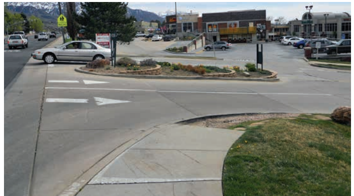
Pedestrian safety and accessibility should not end at the sidewalk, but should extend to building entrances.
