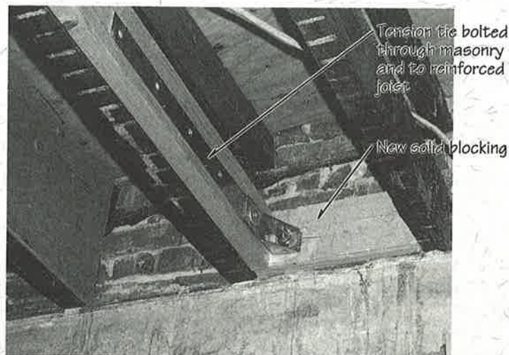
Reinforced Joist/Masonry Wall Connection
