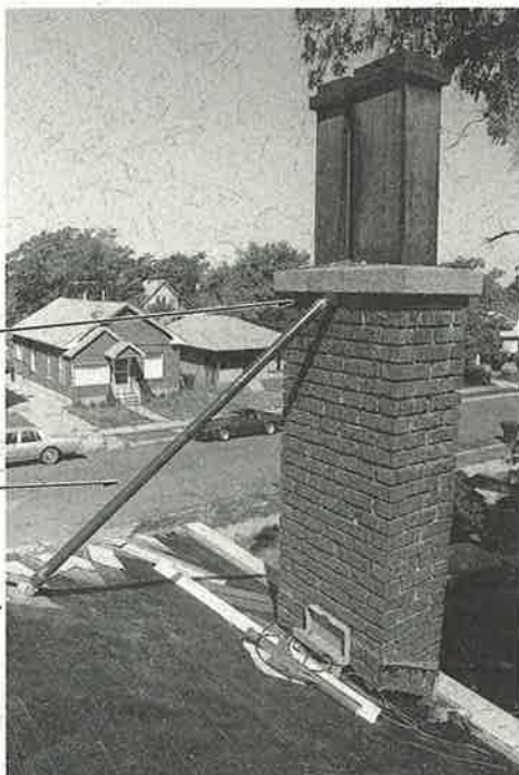
Braced Masonry Chimney
