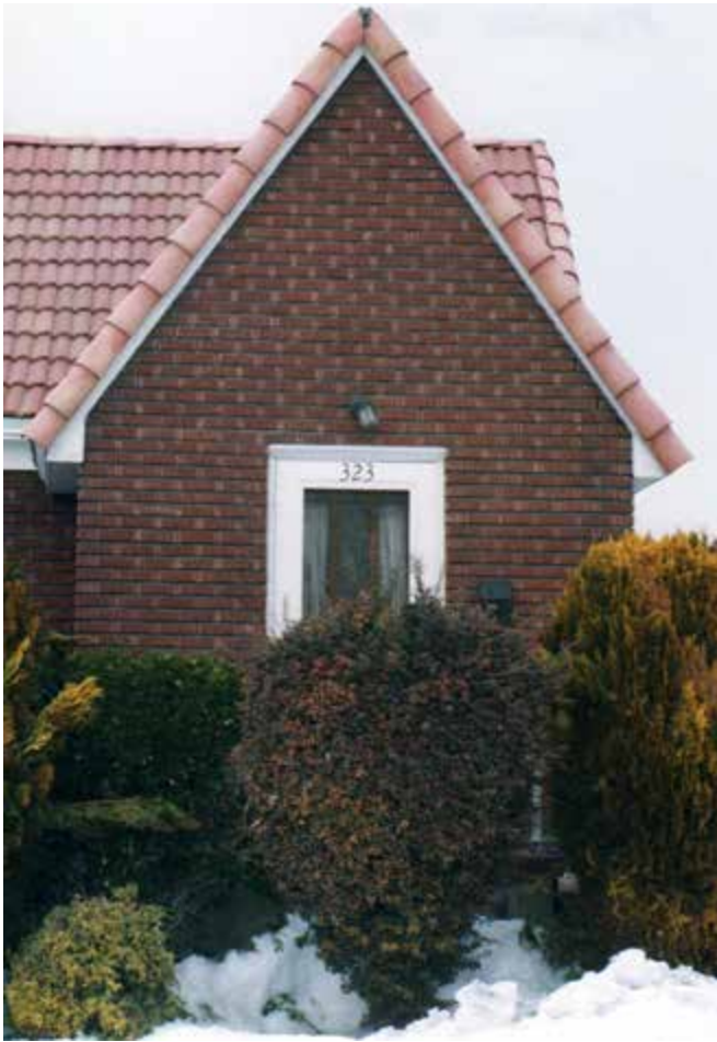
Figure 40. URM gable end walls.
