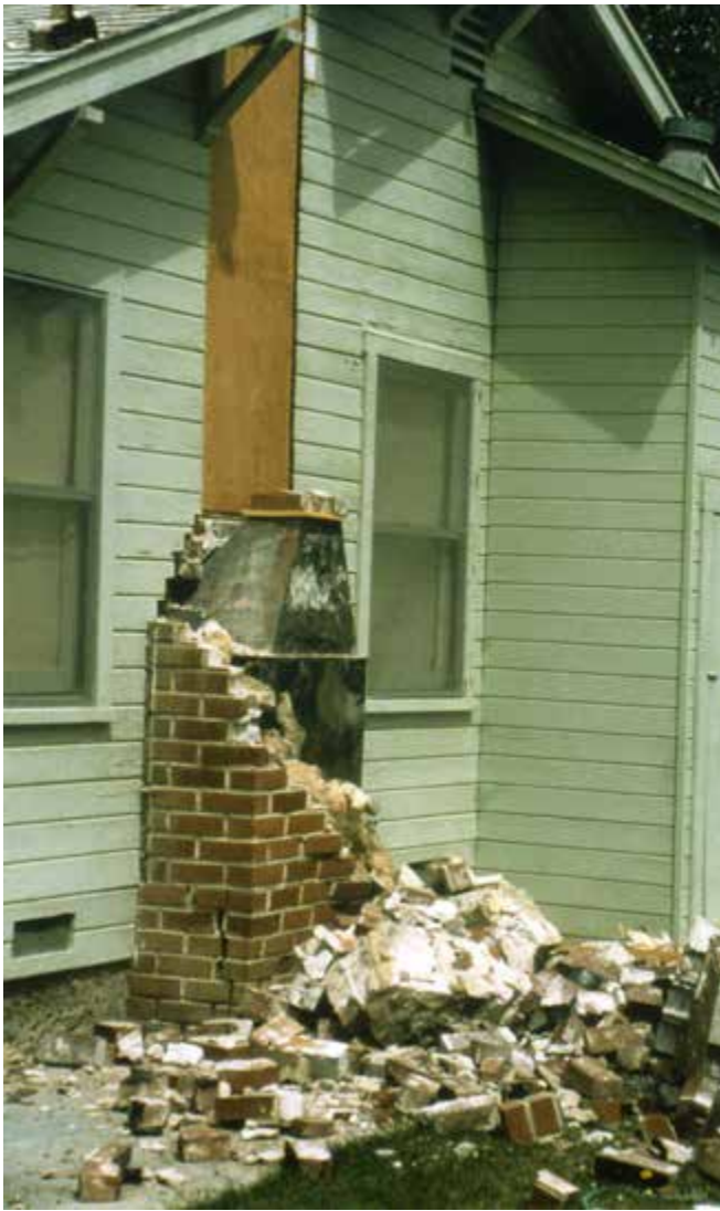
Figure 12. Chimney collapse.
