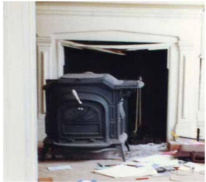
Figure 13. Displacement of wood burning stove.
