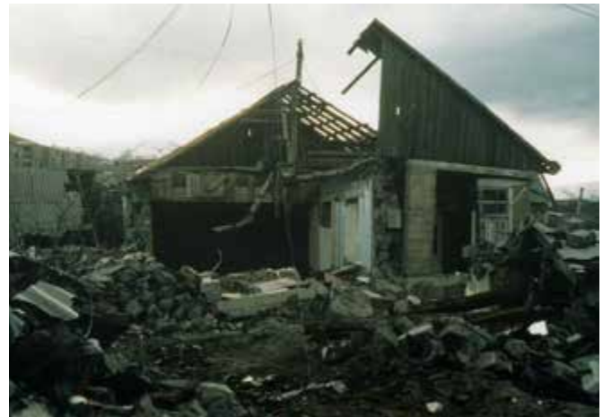
Figure 3. URM structure collapse.
