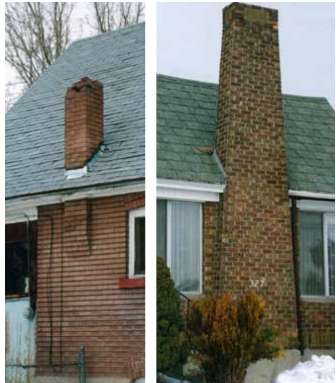
Figure 41. Typical URM chimneys.
