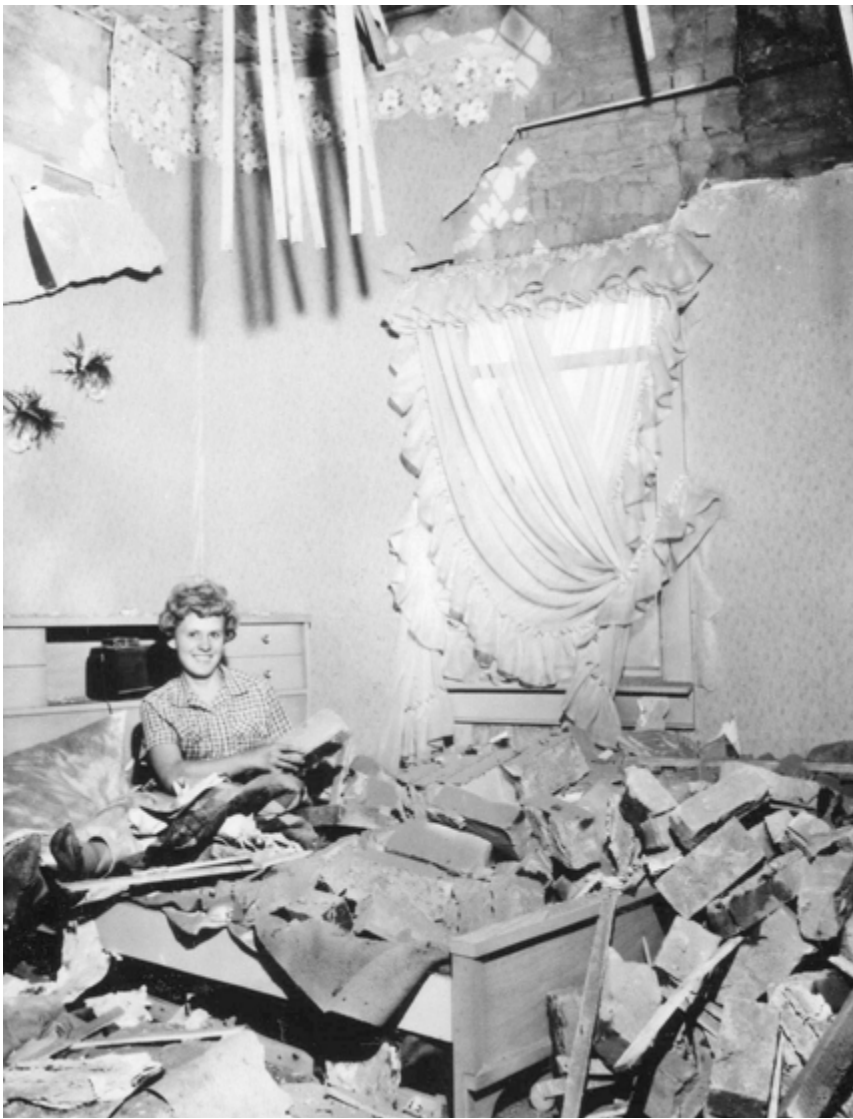
Figure 4. Interior URM wall collapse. Photo: Ariel Benson
