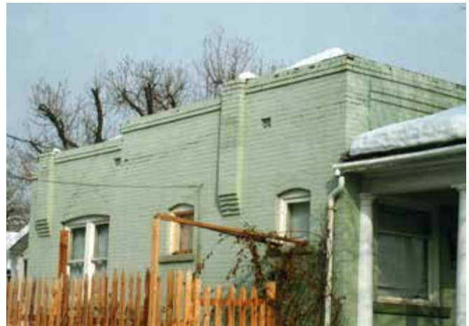
Figure 39. URM parapet walls.
