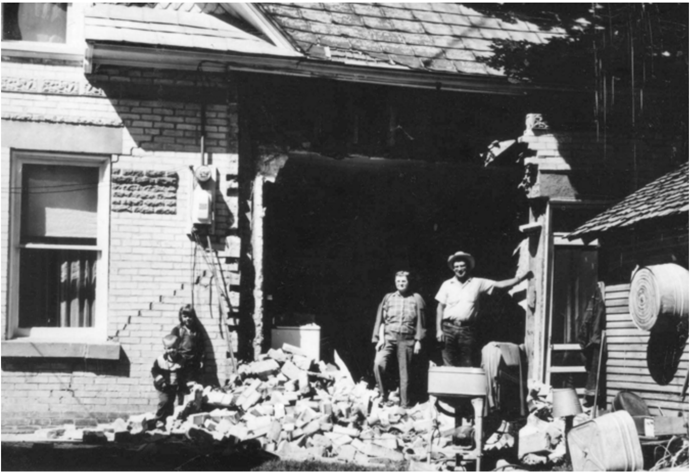
Figure 6. URM wall collapse from earthquake damage. Photo: Ariel Benson
