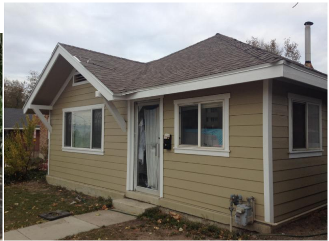
Photo of the south façade post modifications
