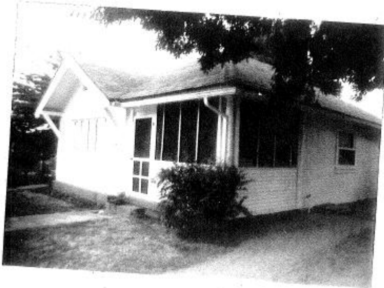
South and East Elevations of 1337 E. 500 S. Photo taken in 1980
