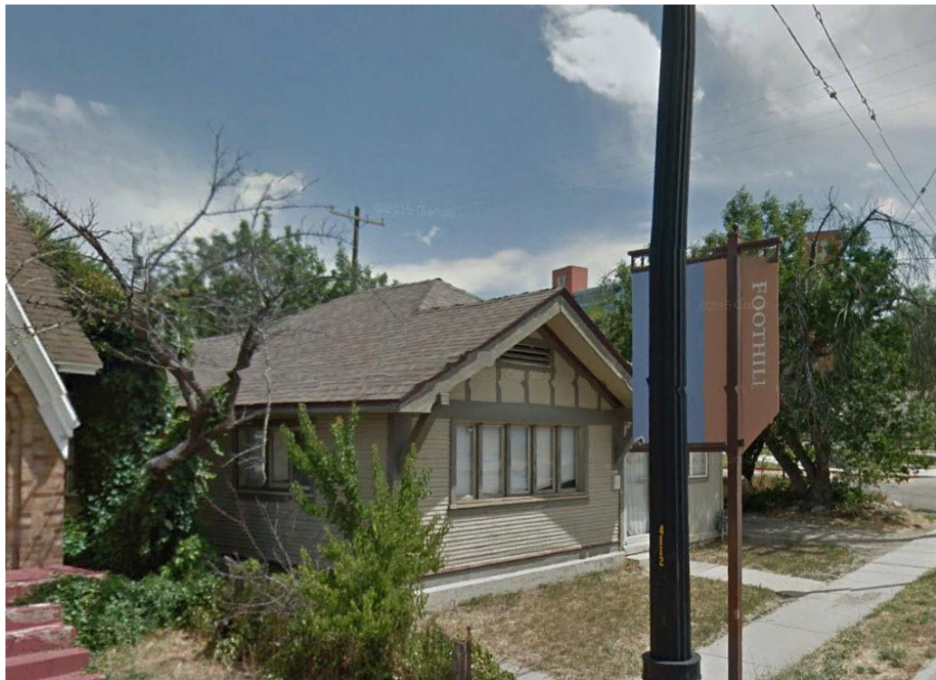
South and portion of West façade, prior to modifications
