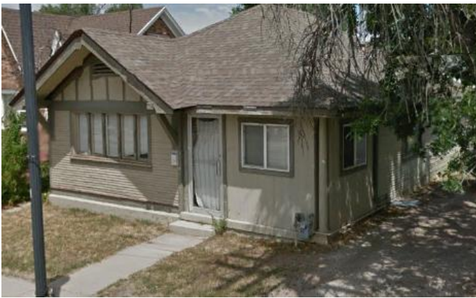
Photo of the south east corner prior modifications
