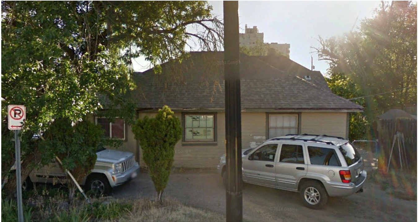
East façade prior to any modifications
