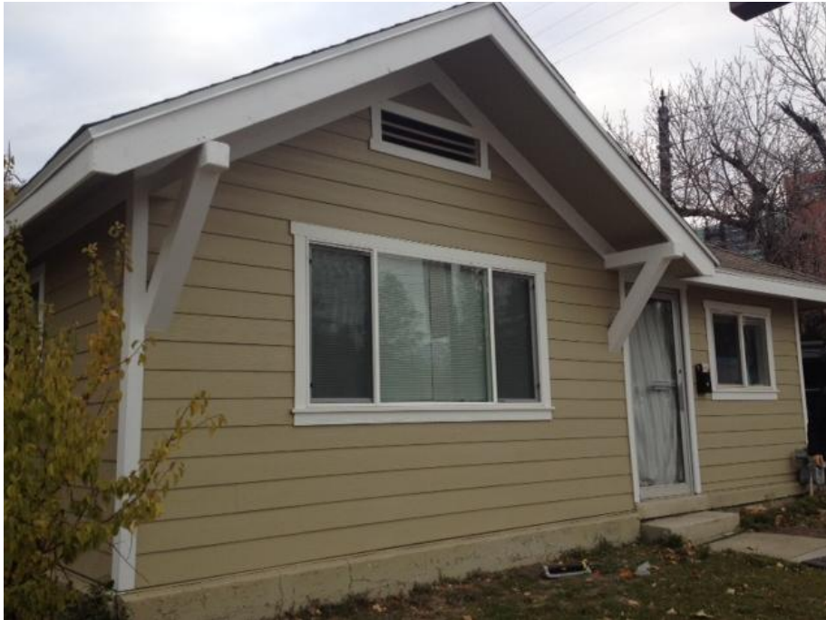
Photo of the recently installed hardy board siding
