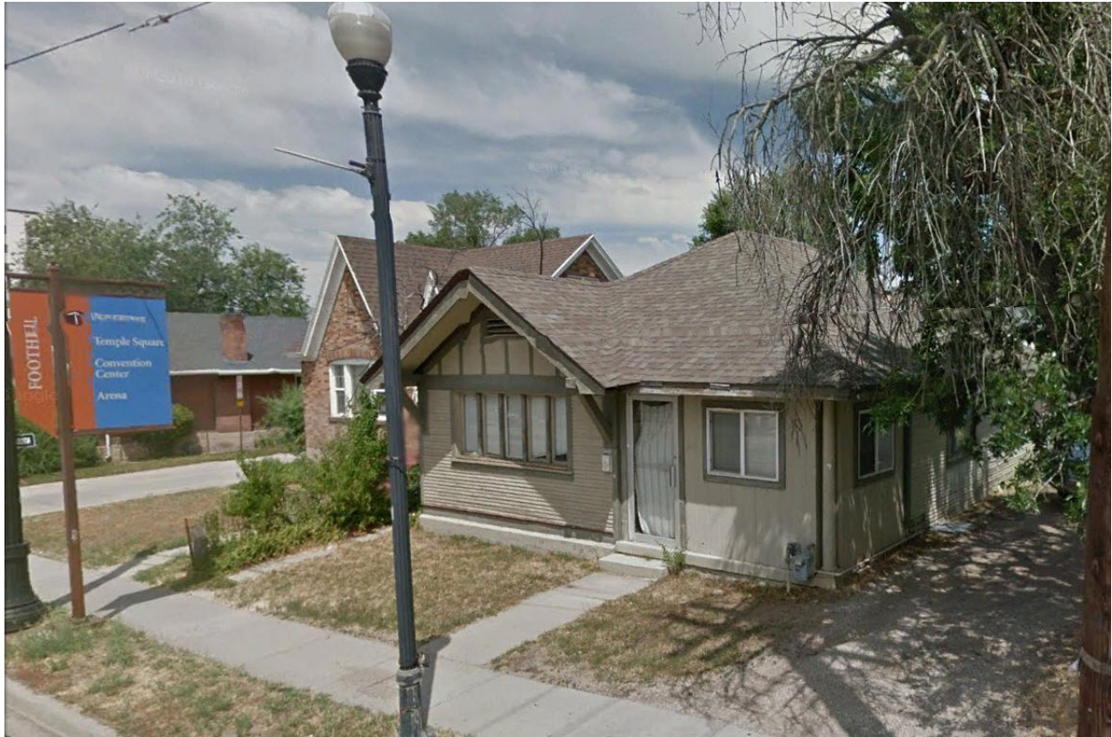
South and portion of the East façade, prior to modifications
