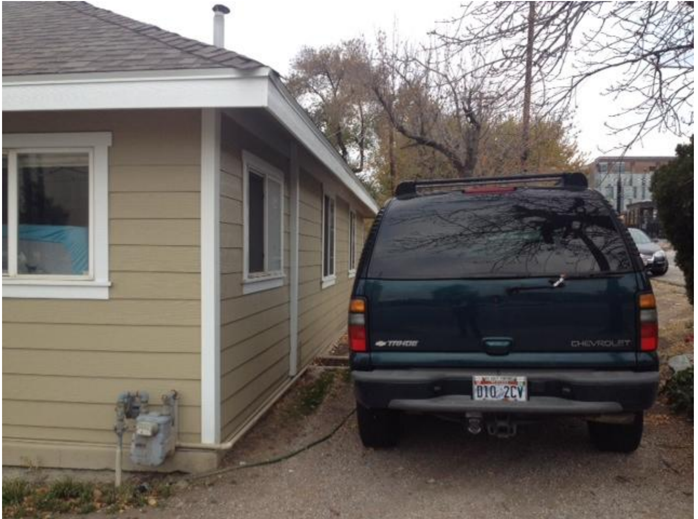
East façade after modifications
