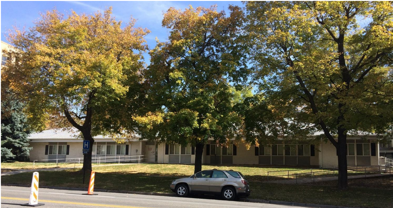
Current conditions-East view of subject property (35 S. 900 E) from 900 East
