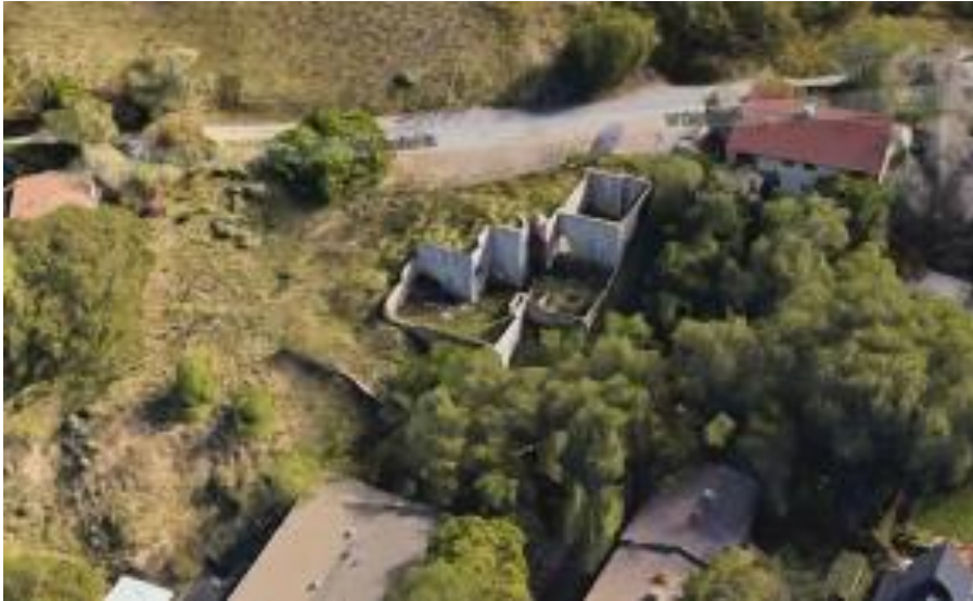
An aerial view of the subject site showing the existing foundation.
