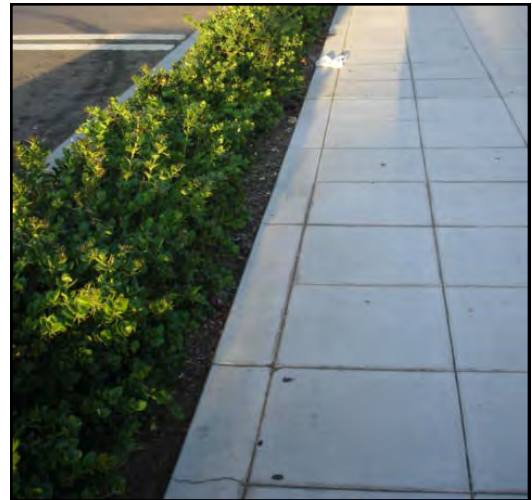
Pedestrian walkways should be separated from drive aisles. This low hedge provides a clear separation.
