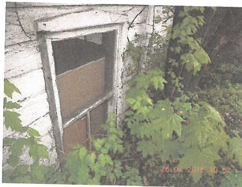
Photo 14 – Retained soils at the north exterior wall
