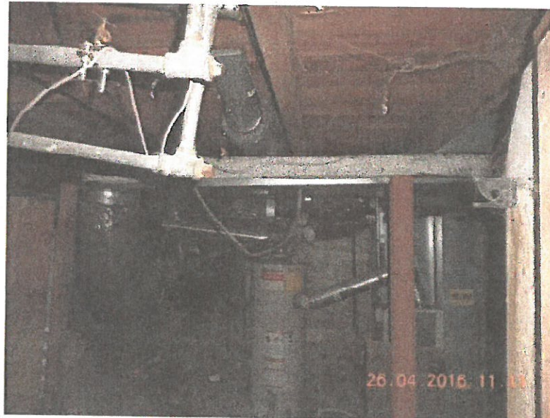
Photo 6 – Apparent added shoring for floor support
