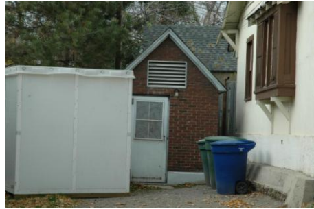
281? N “G” Street (outbuilding)
