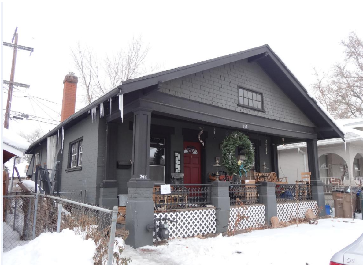
Subject property prior to modifications
