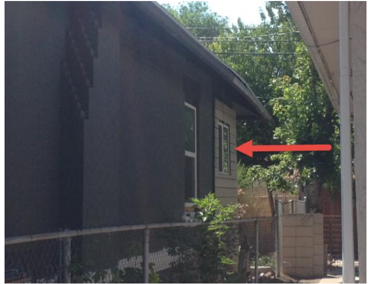
The north elevation post modifications
