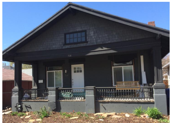
The east elevation post modifications
