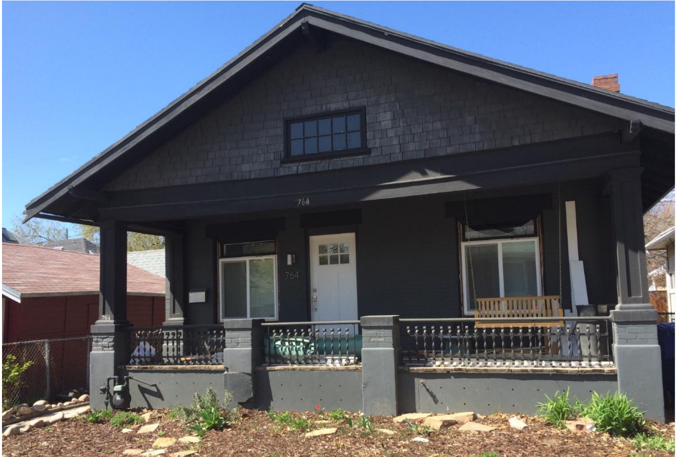
Subject property post modifications
