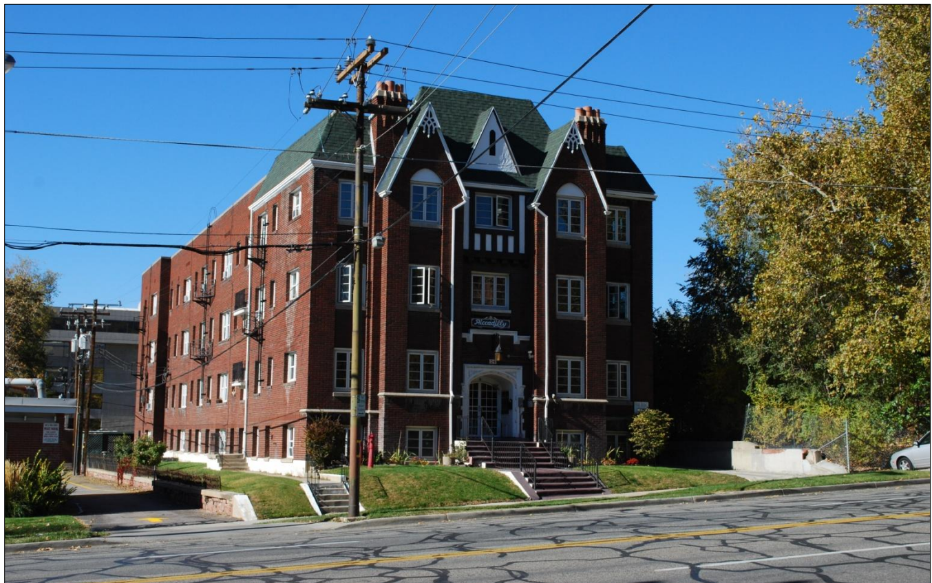
PICCADILLY APARTMENTS, 24 SOUTH 500 EAST
