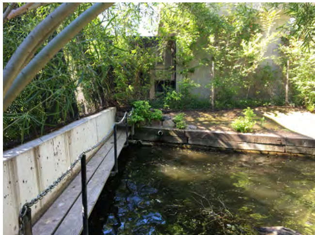
10 Concrete weir at Kennecott Wetlands
