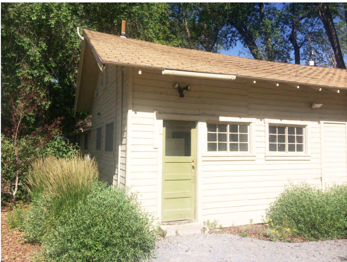
Office house/aquarium structure. Photo taken from relatively the same angle as historic photo above. West portion of the structure can be seen in the photo.
