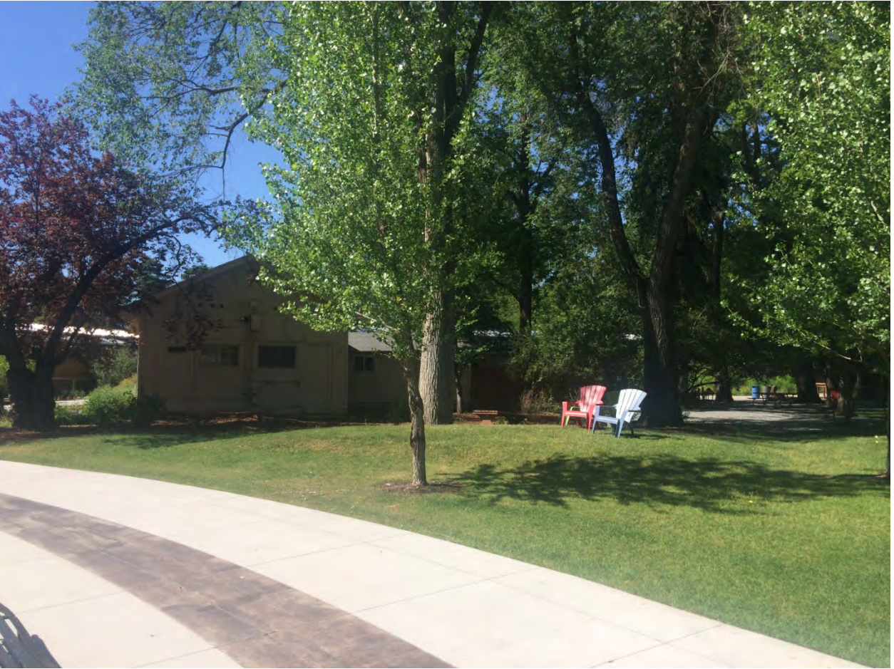
View of office house/aquarium building (north elevation) as seen from the pedestrian path near Tracy Aviary's main entrance
