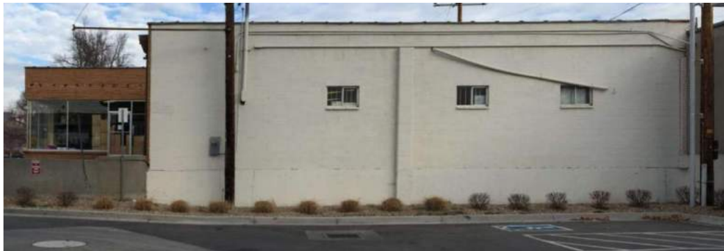
Existing South Façade
