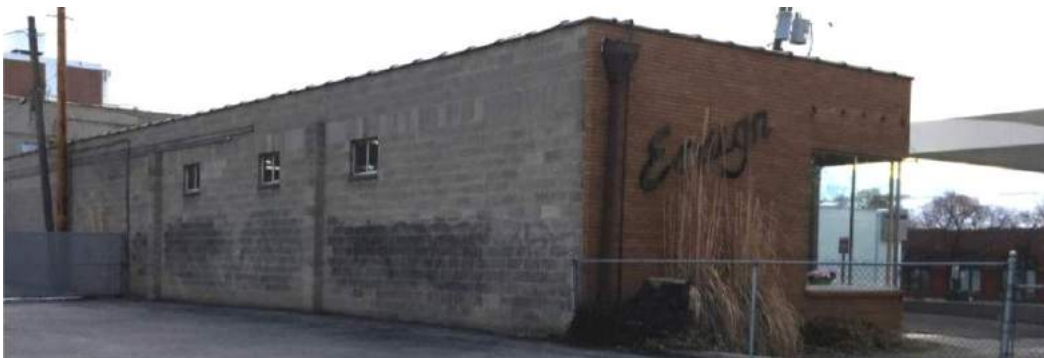
Existing North Façade
