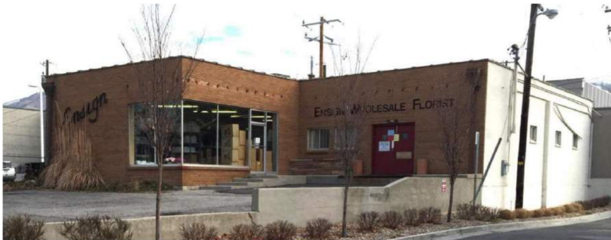
Existing West Facade
