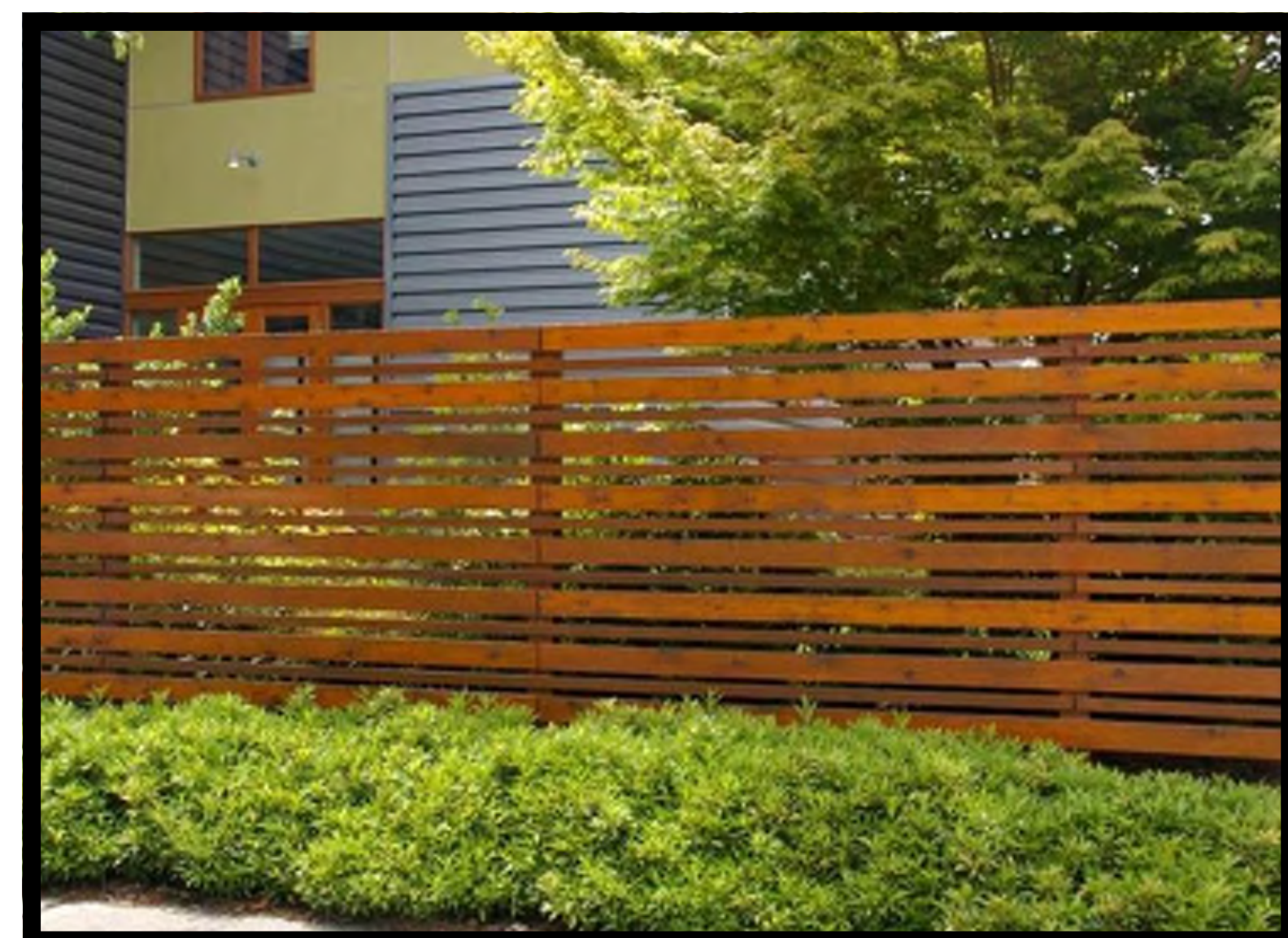
COURTYARD/PATIO RAIL/FENCE 6'-0" SPACING OF MEMBERS WILL VARY BASED ON APPROPRIATE PRIVACY MEASURES DICTATED BY SITUATION
