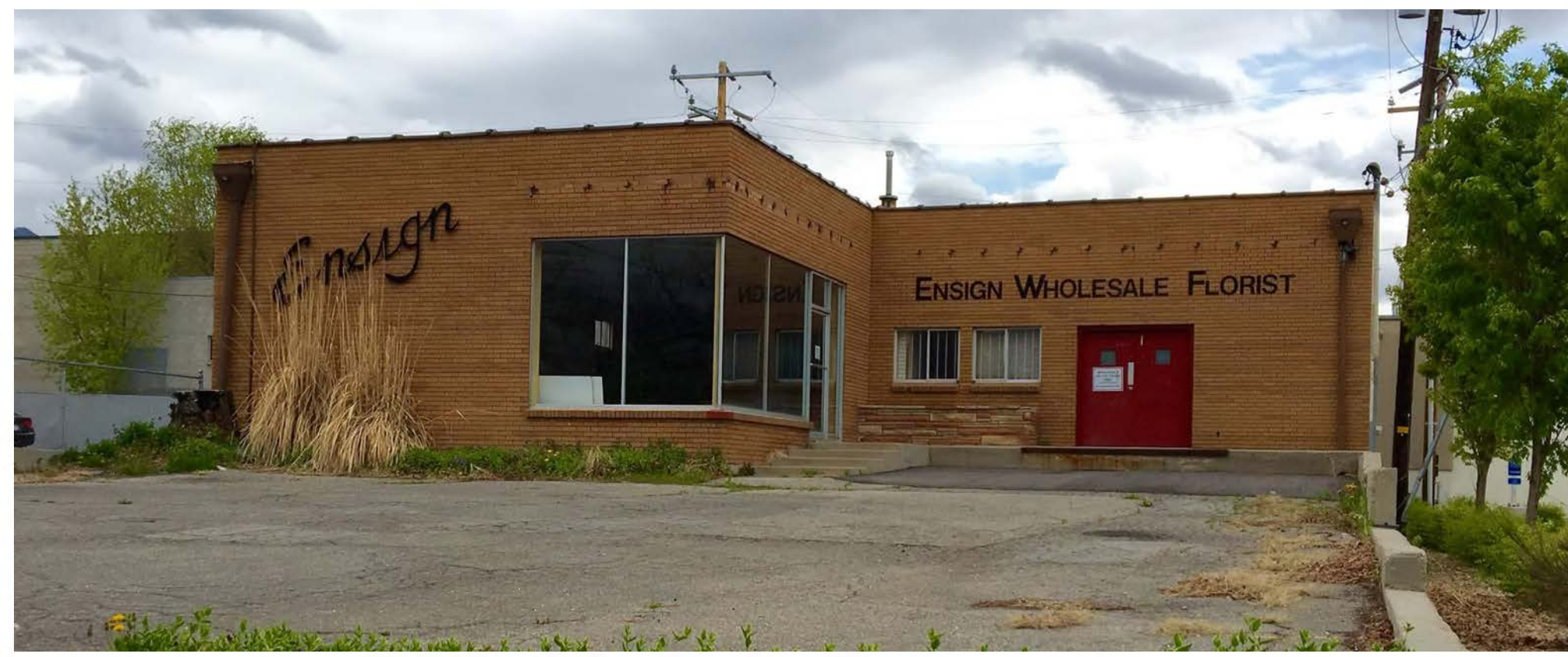
EXISTING WEST FACADE
