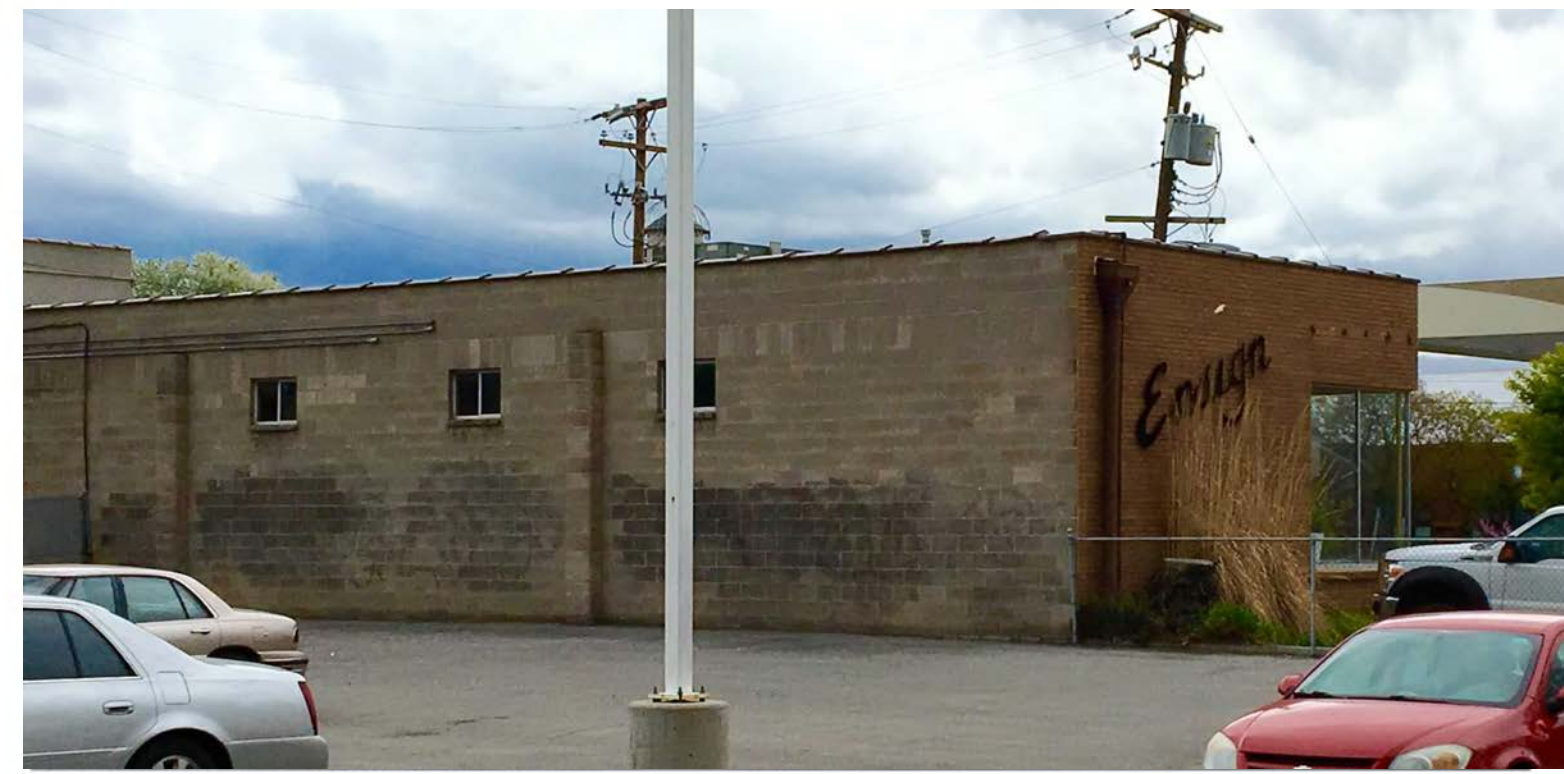
EXISTING NORTH FACADE
