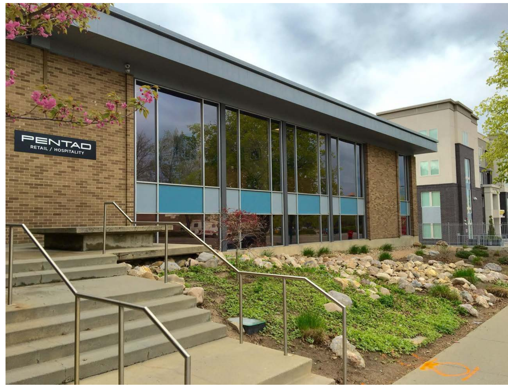
2 - OFFICE BUILDING: 560 E 500 S
