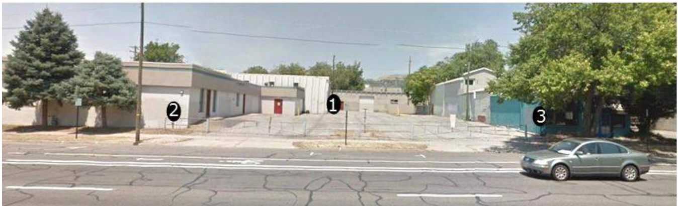
Existing Buildings Proposed for Demolition
