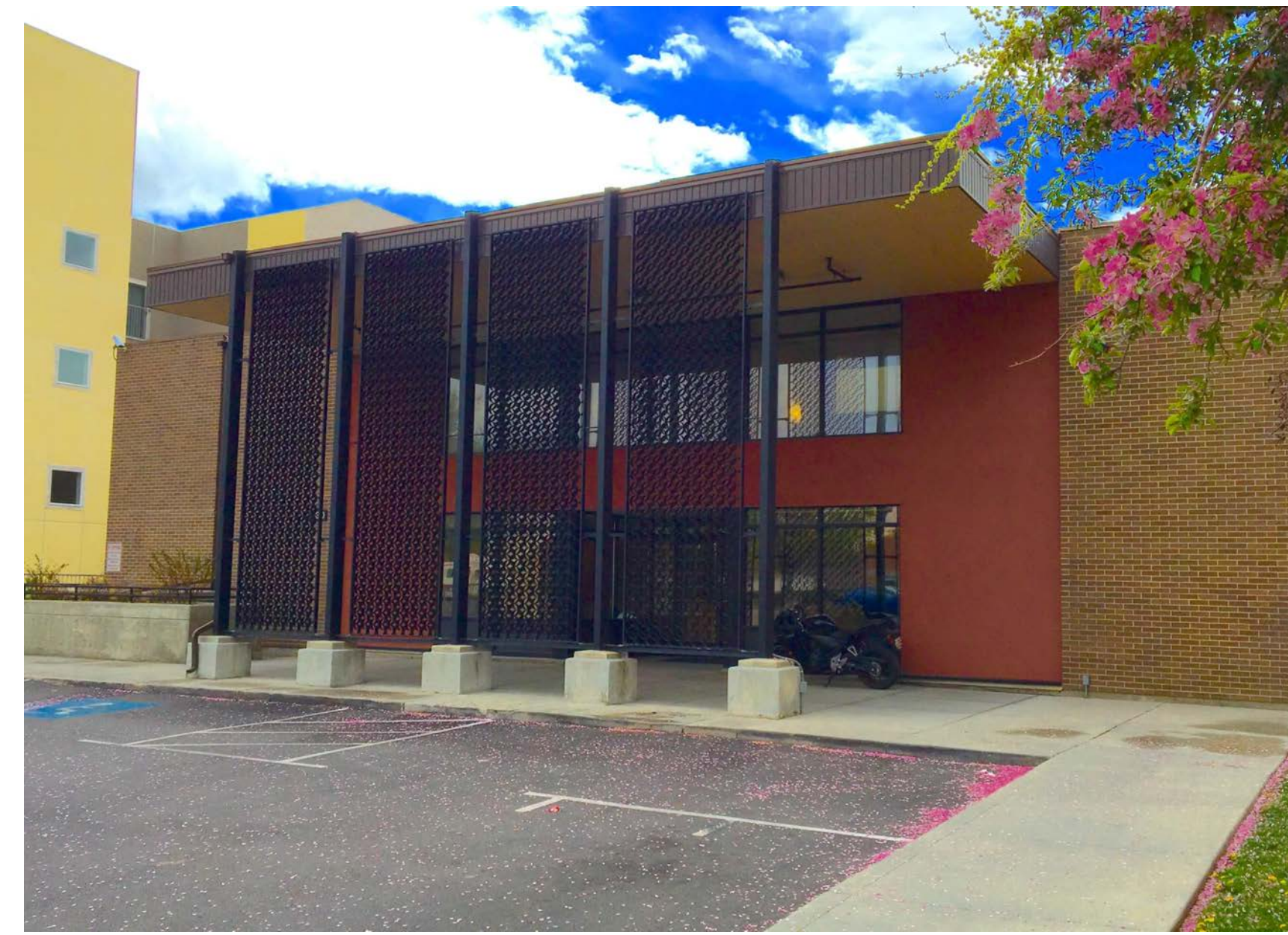
3 - OFFICE BUILDING: 530 E 500 S
