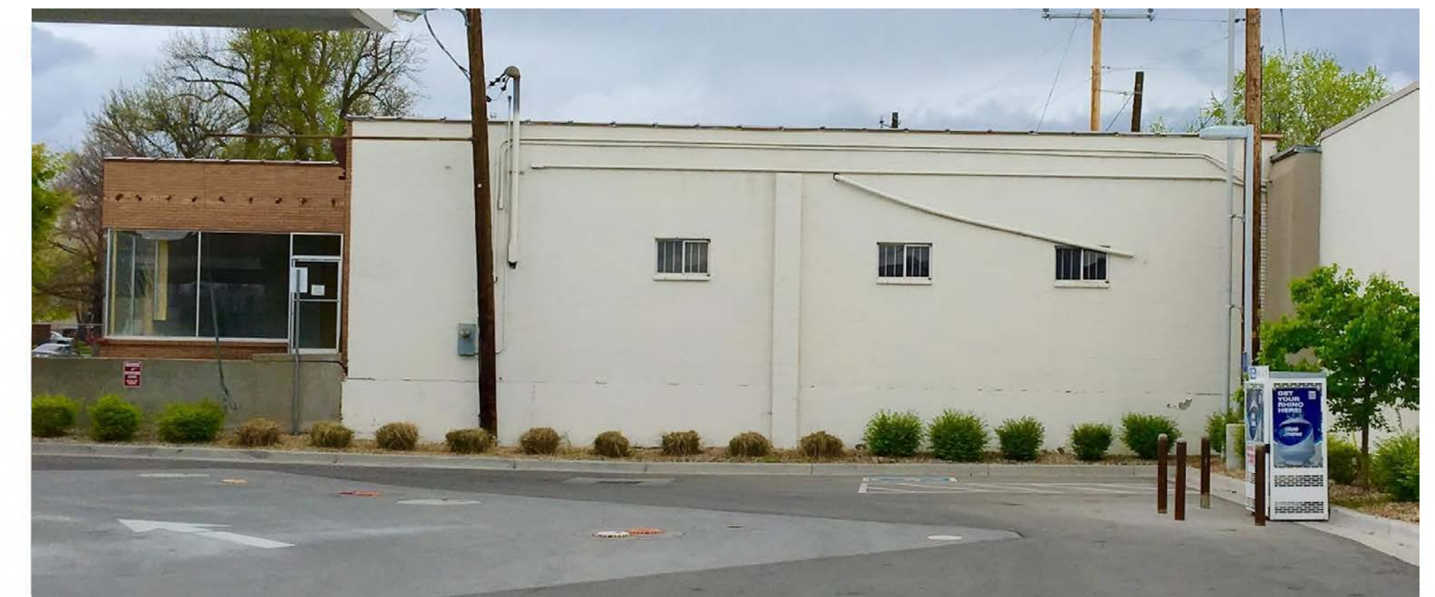
EXISTING SOUTH FACADE
