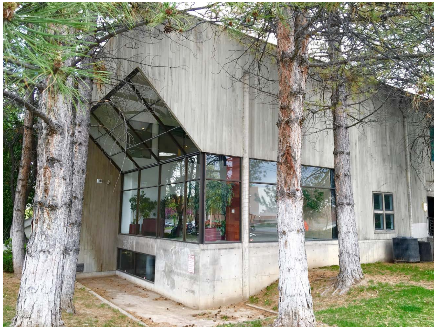
3 - OFFICE BUILDING: 510 S 600 W
