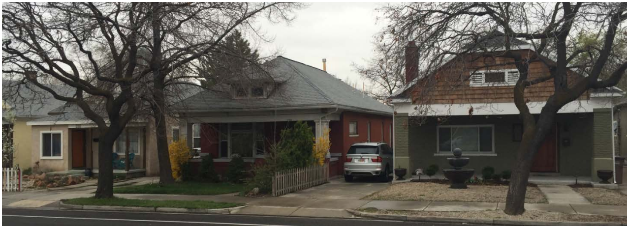
730-726 S 700 E - North of Site
