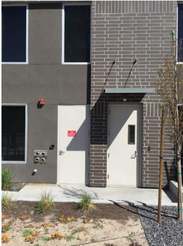
Images like these show utilities and backexit doors located on the principle street elevation of buildings throughout the city. This lack of attention to detail says to the pedestrian and the public in general that the building has turned its back to the public realm.
