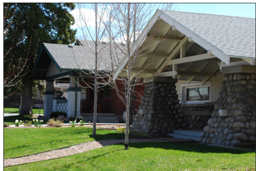
A concentration of bungalow designs typifies the earliest phase of development in Westmoreland Place.
