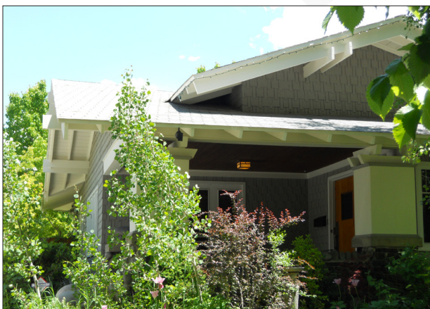
Horizontal lines and low roof profiles are characteristic of the Craftsman style bungalow and prompt designing an addition within and behind these profiles.
