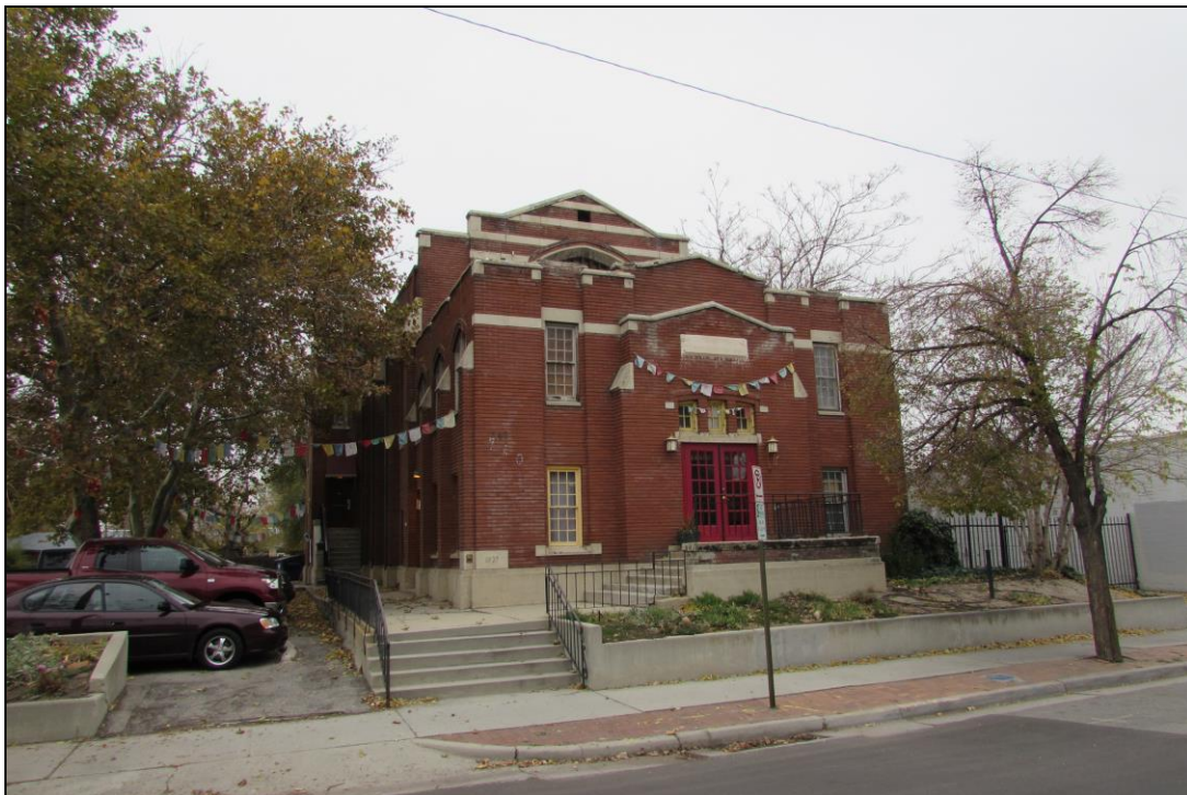
Photograph 14 of 25: LDS Fifth Ward Chapel; 740 S. 300 W.; camera facing northwest
