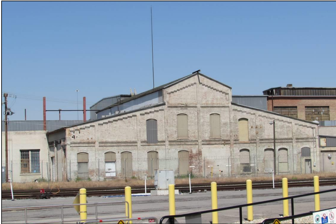
Photograph 7 of 25: D&RGW Boiler House; camera facing west
