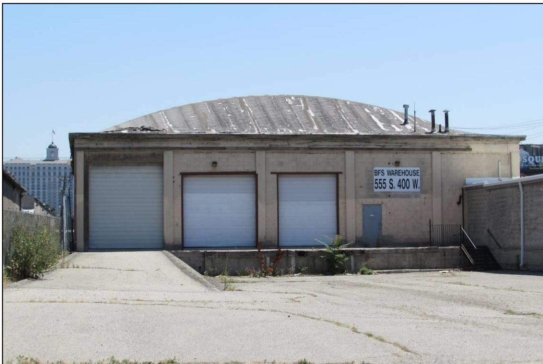
Photograph 20 of 25: Drive-up warehouse; 555 S. 400 W.; camera facing east
