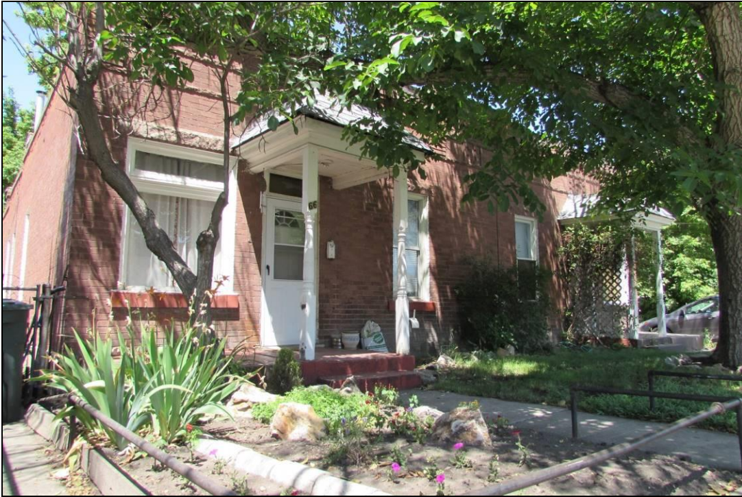
Photograph 5 of 25: Example of 1869-1899 period duplex dwelling; 64-66 S. 600 W.; camera facing northwest
