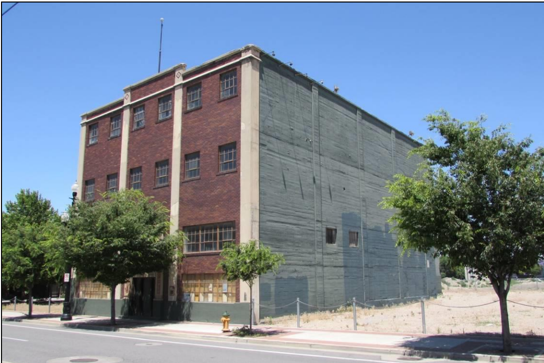
Photograph 16 of 25: Central Warehouse; 520 W. 200 S.; camera facing northwest
