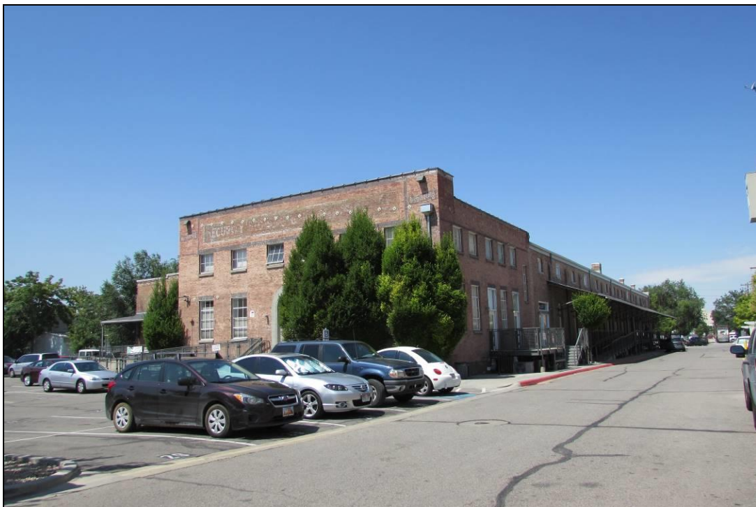
Photograph 8 of 25: Example of 1900-1929 era warehouse; 230 S. 500 W.; camera facing southwest
