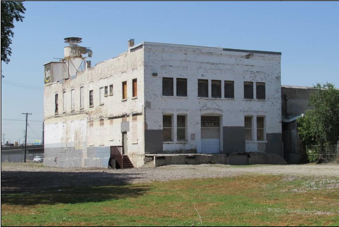
Photograph 17 of 25: Serta Warehouse; 535 W. 300 S.; camera facing southwest
