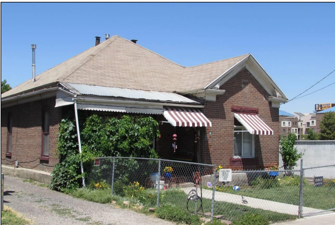
Photograph 6 of 25: Example of 1869-1899 period duplex dwelling; 42 S. 600 W.; camera facing northwest
