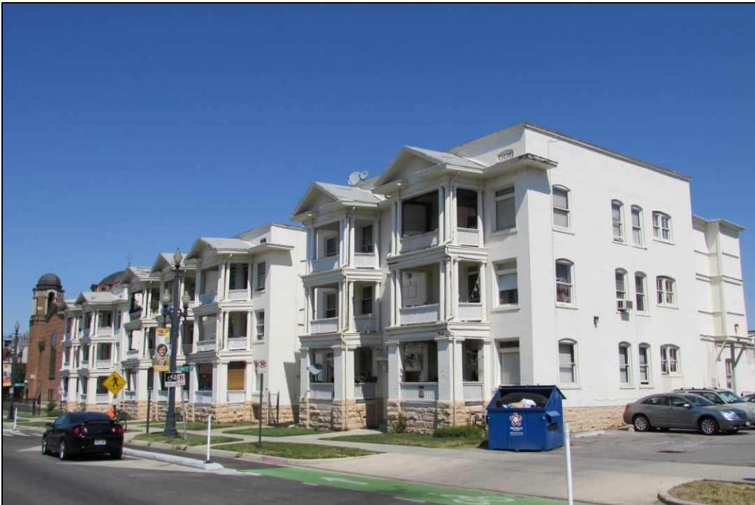
Photograph 10 of 25: Covey Flats/La France walk-up apartments; camera facing northwest.
