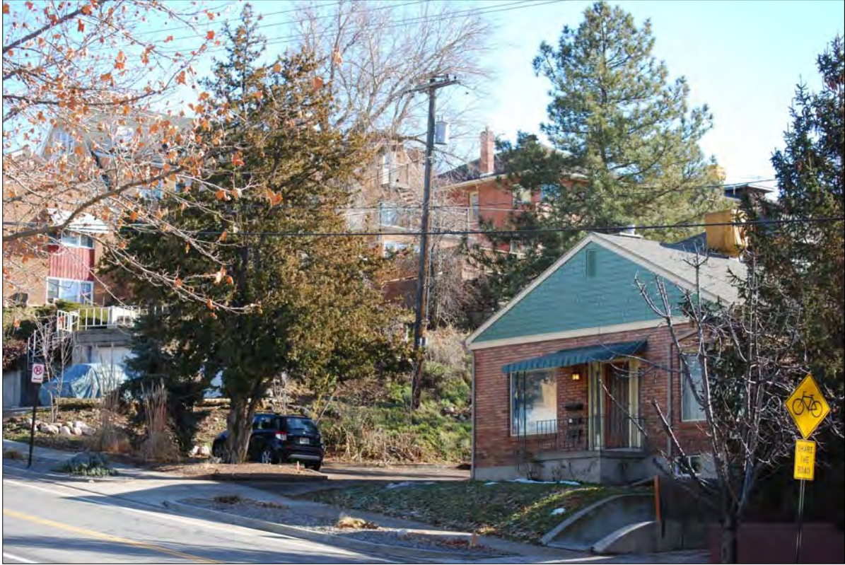
1160 EAST 200 SOUTH - SITE FROM THE WEST
