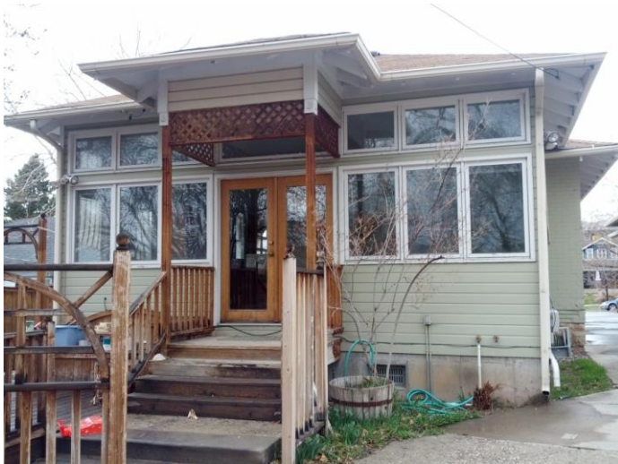
Former rear addition
