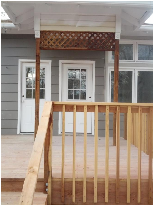
New deck railing and balusters
