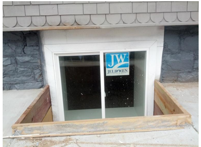
3 New sliding basement windows installed
