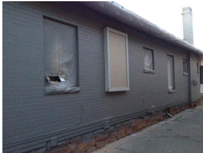
Covered window on east elevation
