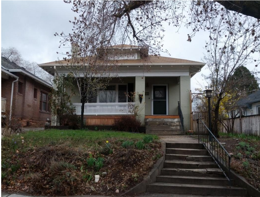
Front of home before concrete work
