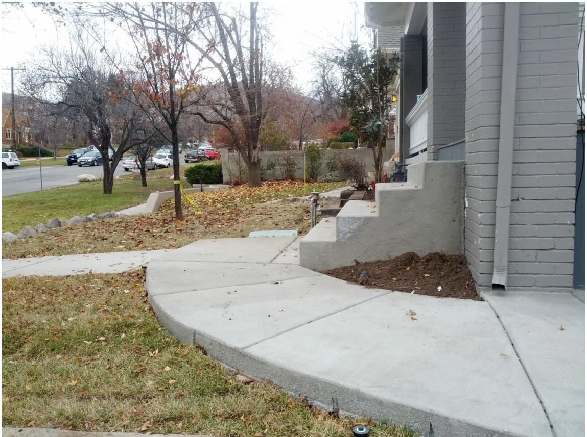
Concrete work and repairs on walkway
