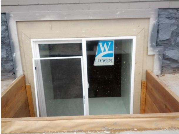
Sliding vinyl basement windows and redwood window wells that were installed.
