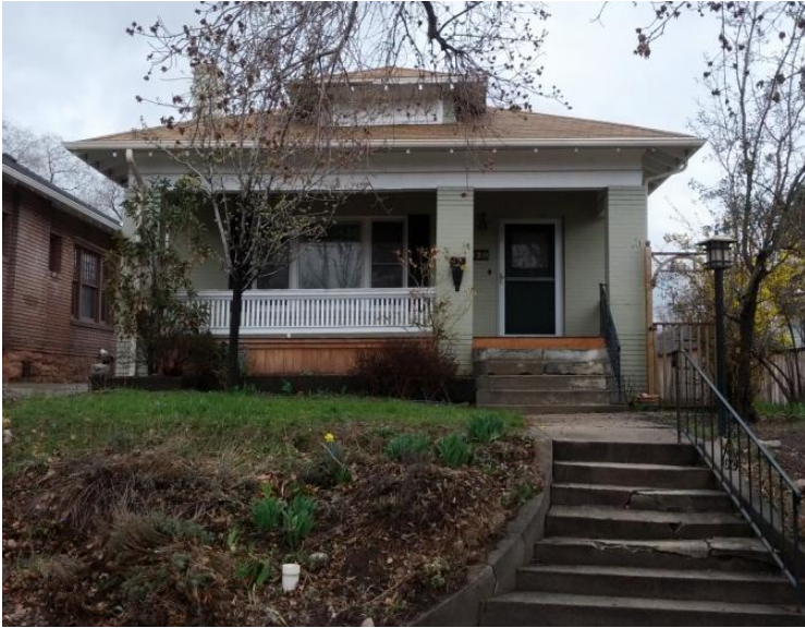
Former front porch and front yard handrails
