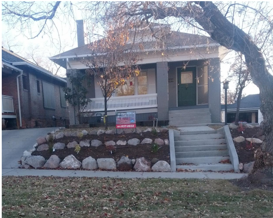
Front of home after concrete work
