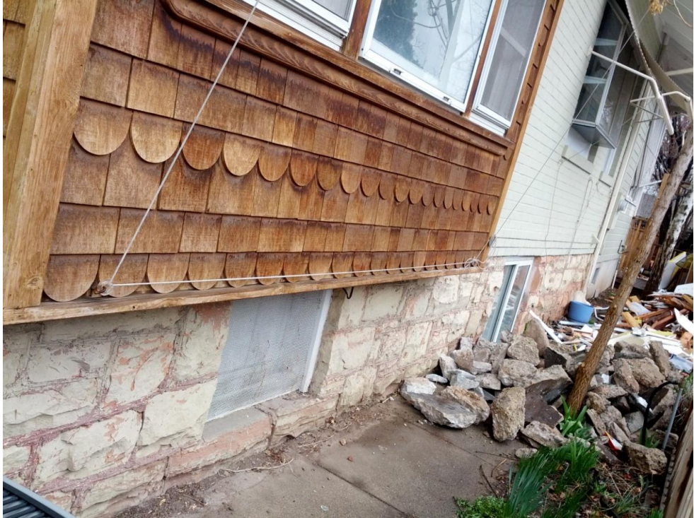
Original sandstone foundation
