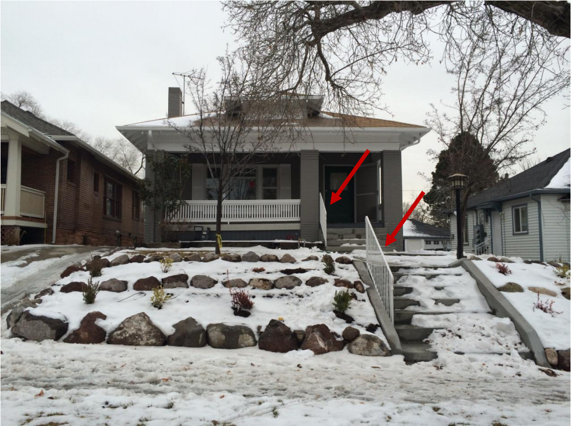
New front painted metal handrails (below)
