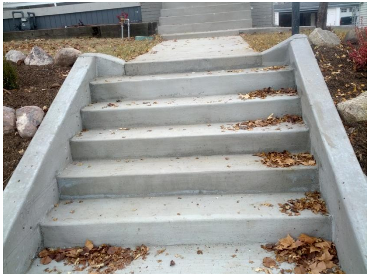
New design of front stairs
