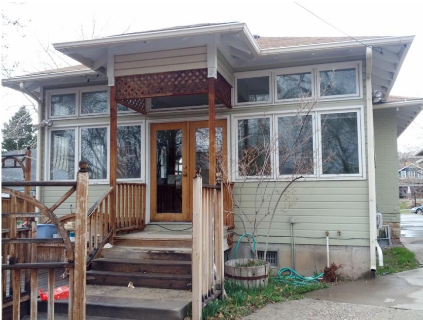
Former rear addition/porch
