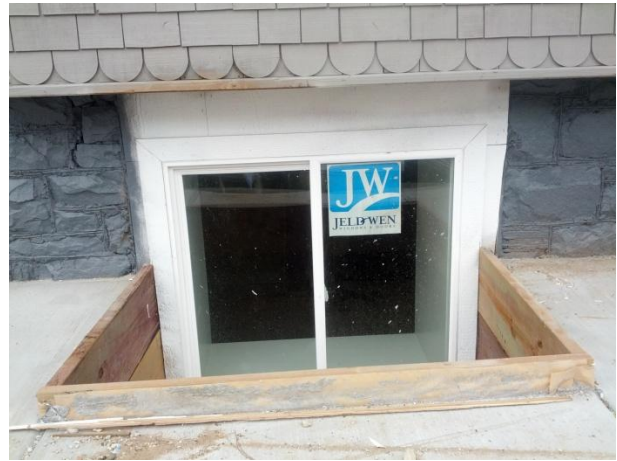
Sliding vinyl basement windows and redwood window wells that were installed.
