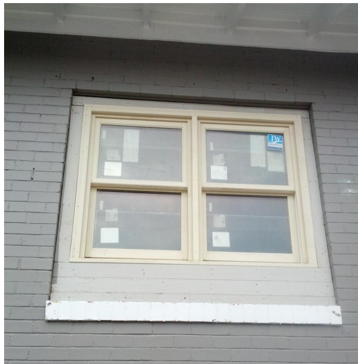
New wood double hung kitchen replacement windows
