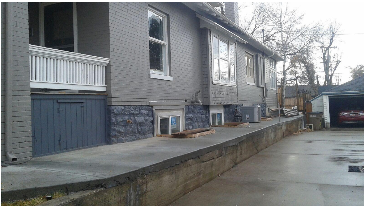
Concrete work along western edge of property
