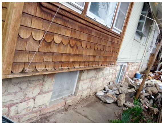
Basement windows before alterations
