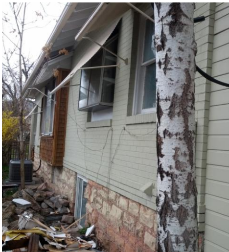
Former garden box kitchen window
