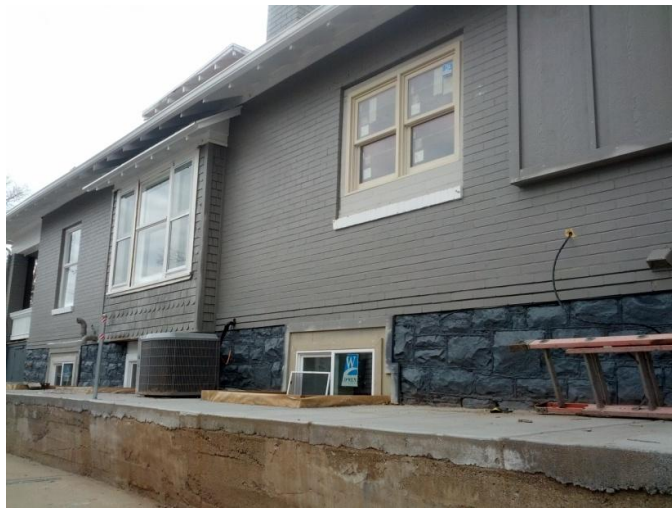
New kitchen window and covered window on west elevation
