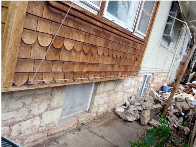
Former Basement Windows – West Elevation
