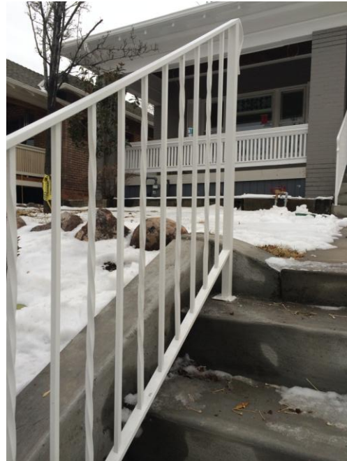
Newly installed handrails
