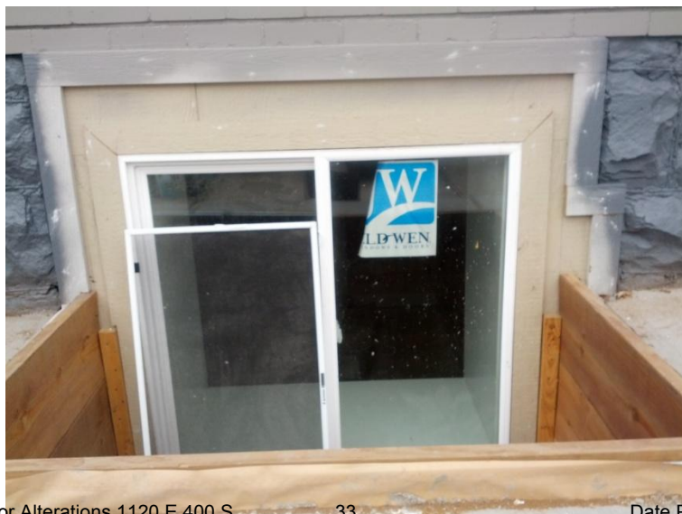
3 New sliding basement windows installed
