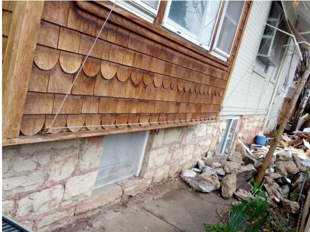
Unpainted original sandstone foundation
