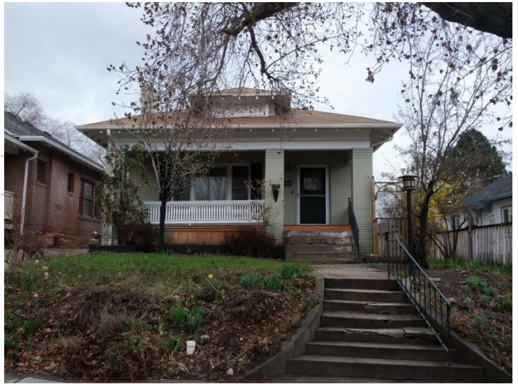
Stairs and walkway prior to concrete work
