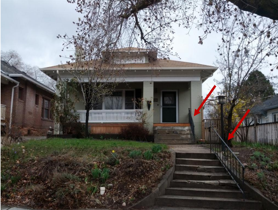
Former front metal handrails along front porch and front yard (above)
