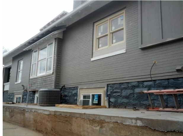
Original sandstone foundation was painted dark gray
