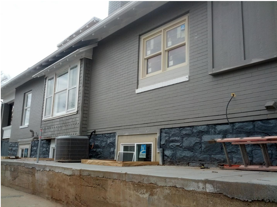
Original sandstone foundation painted dark gray
