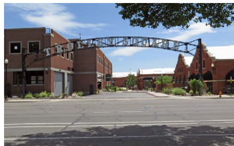
pole sign (pad site A)
