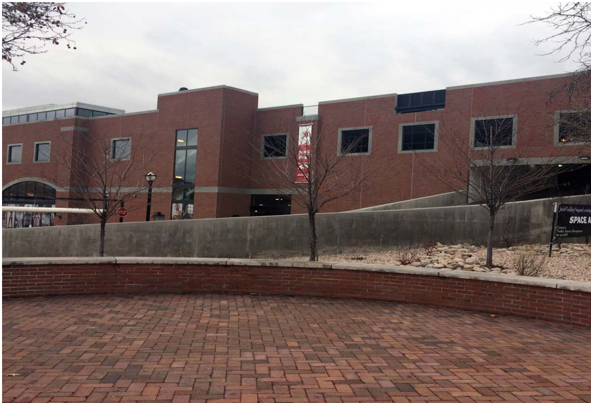
View of northeast corner of the site where the shopping center identification pole sign with an internally illuminated electronic changeable copy panel is proposed. The proposed location just behind the brick wall is approximately 3' above sidewalk grade. The proposed 18' 9" sign would have a height of 21' 9" above sidewalk grade. Scale and height of the sign should be consistent with the character of the site.
