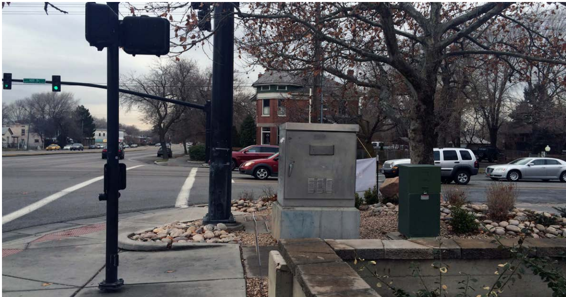
View of proposed location for the monument sign looking south. Wall will be reconstructed to a curved shape.
