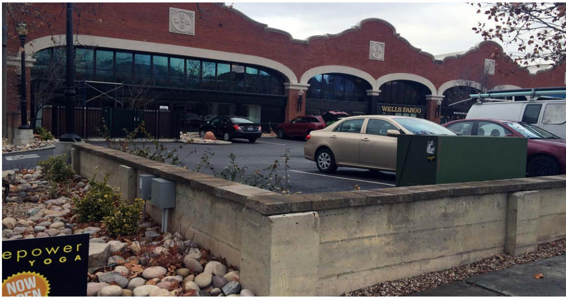
Proposed location of Monument sign on 600 South and 700 East. The proposed height of the monument sign (7' sign + 3' base) and 14' wide would visually block views of the historic architecture.
