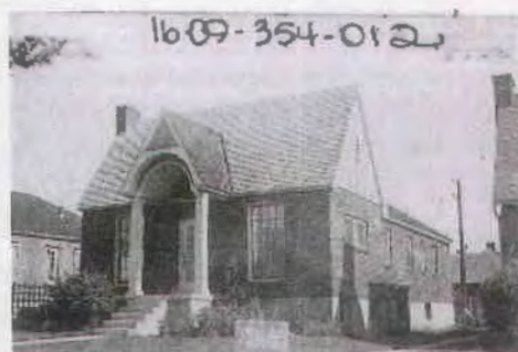
1392 E. Laird Ave Built : 1927 Neoclassical/English cottage
