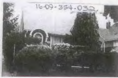
1355 E. 1300 South Built : 1926 English Cottage
