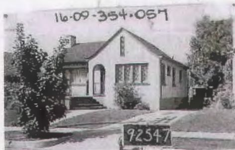
1224 S. 1500 E. Built: 1925 Late 20th Century
