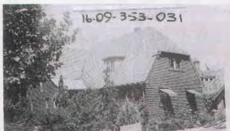
1347 E. Laird Ave. Built : 1926 English Cottage
