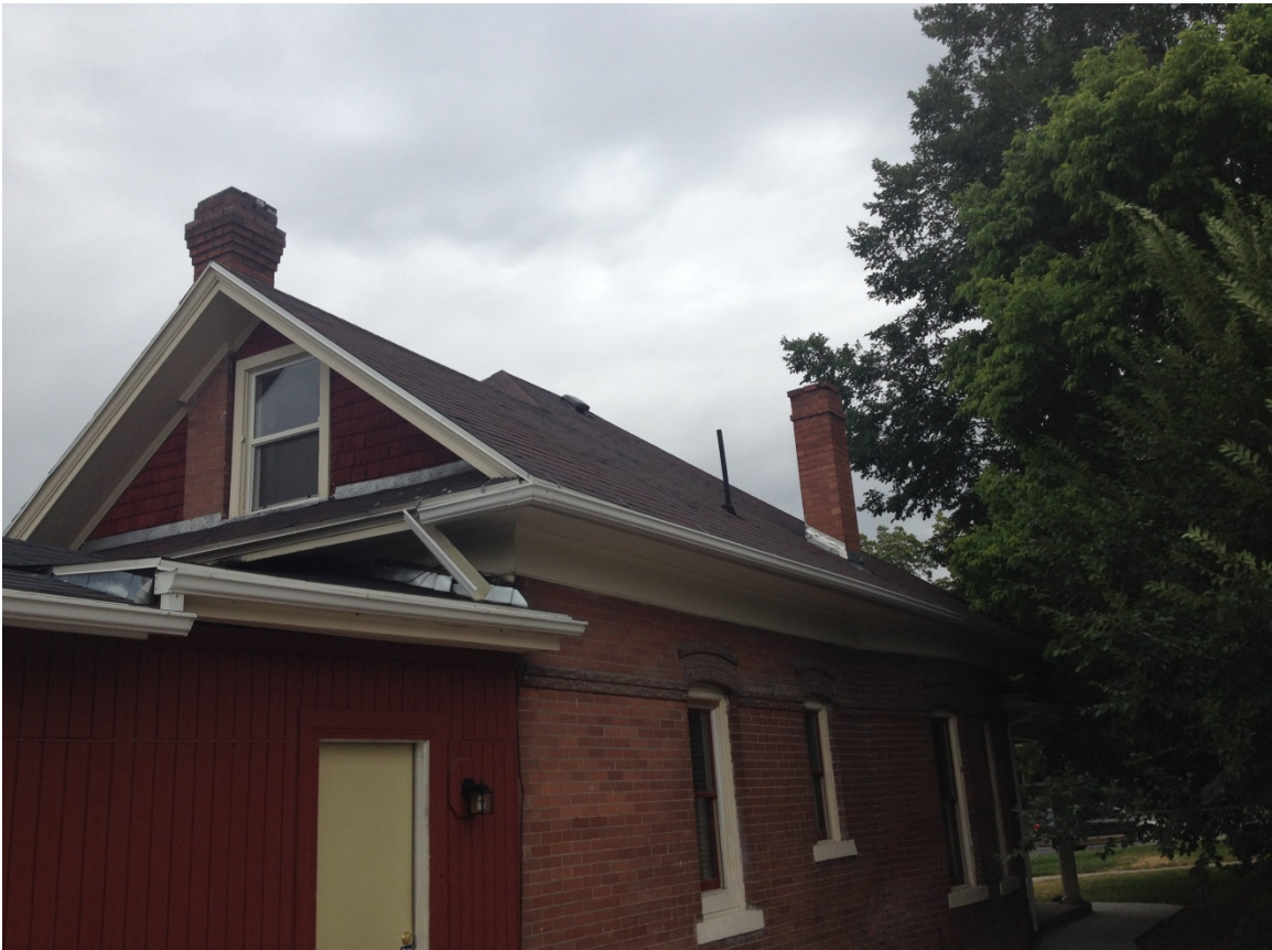
Chimneys to be Removed
