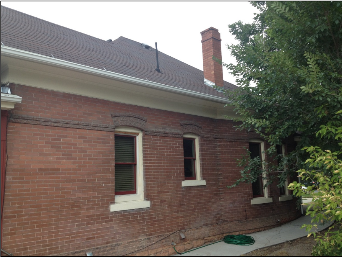
Northern Chimney to be Removed
