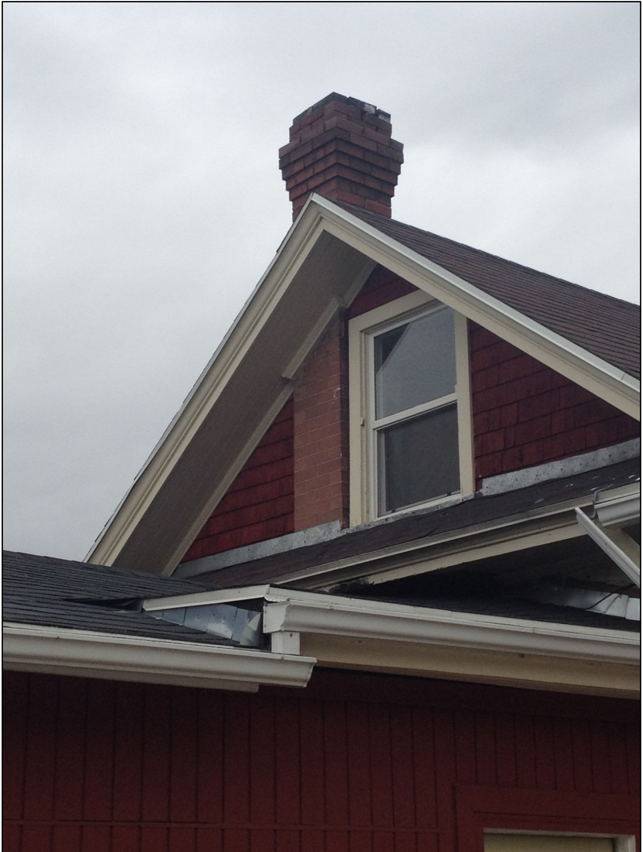
Southern Chimney to be Removed
