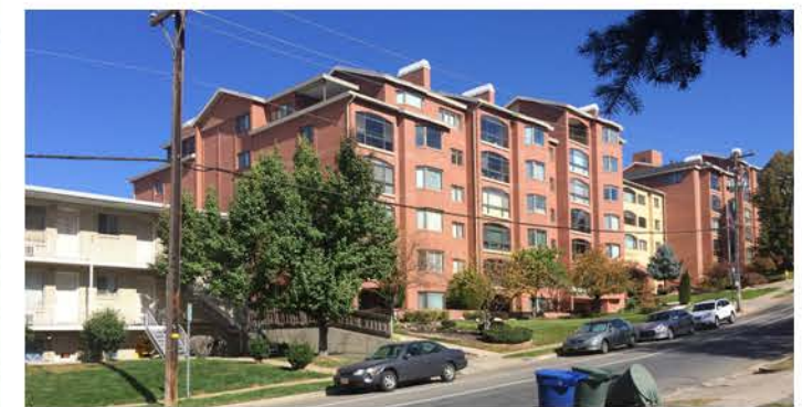
④ View from 138 E. 3rd Avenue
