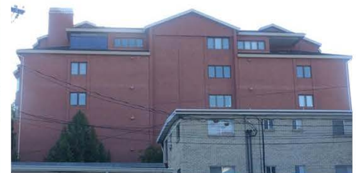
③ View from the rear of 131 E. 3rd Avenue
