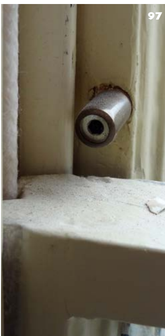
97: Height restrainers allow a degree of ventilation without compromising security.
