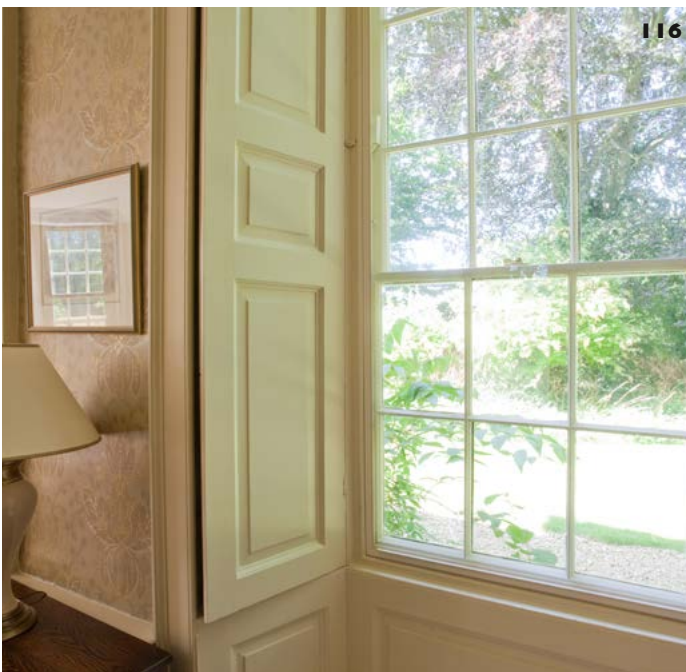
115: Failing plastic coated aluminium double glazed windows to this listed terrace house were replaced with single glazed timber casements to the correct historic pattern with secondary glazing incorporating Low E glazing giving a centre pane U-value of 1.6w/m 2 K.
