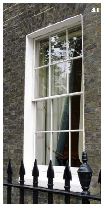
41: In 1774, further legislation in London led to sash boxes being hidden within a rebate formed in the brickwork surrounding the window opening. This, combined with very slender glazing bars gave windows a much lighter and more delicate appearance.
