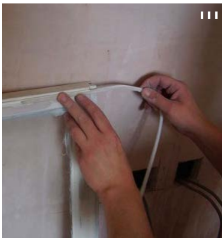
111: Nylon brushes being inserted into the sash as draught-proofing.
