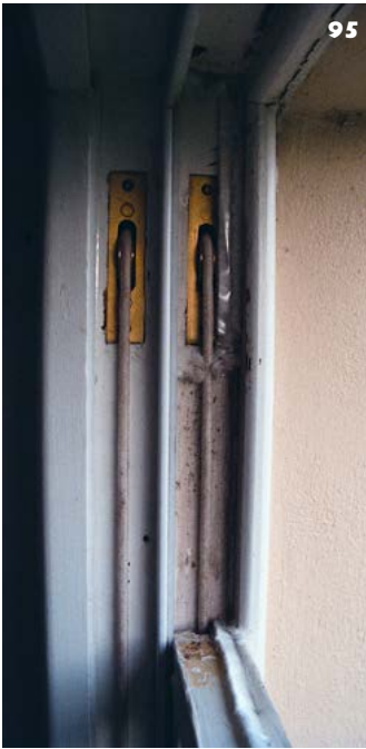
95: In a double hung sliding sash window each sash has its own pulley and cord. The parting bead separates the sashes and holds them in position. The cord and pulley need to be kept in good working order.
