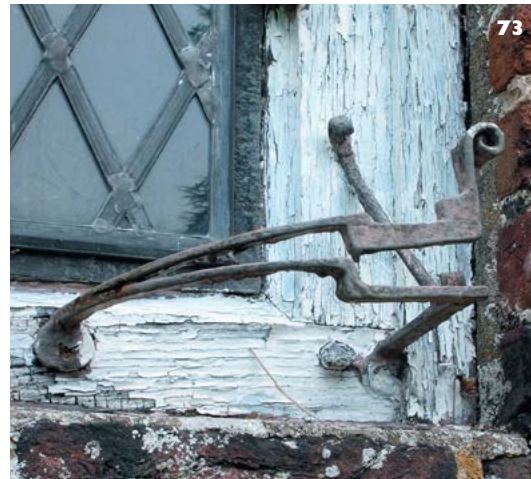
66: A window hinge made up of a pintle and gudgeon.
