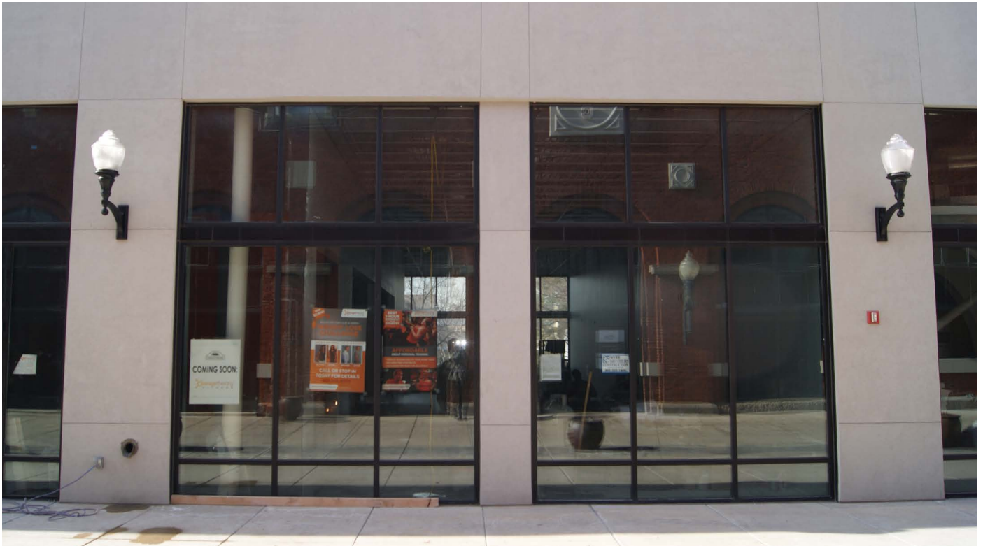
East elevation of the Orange Theory Fitness lease space where one of the signs is proposed.
