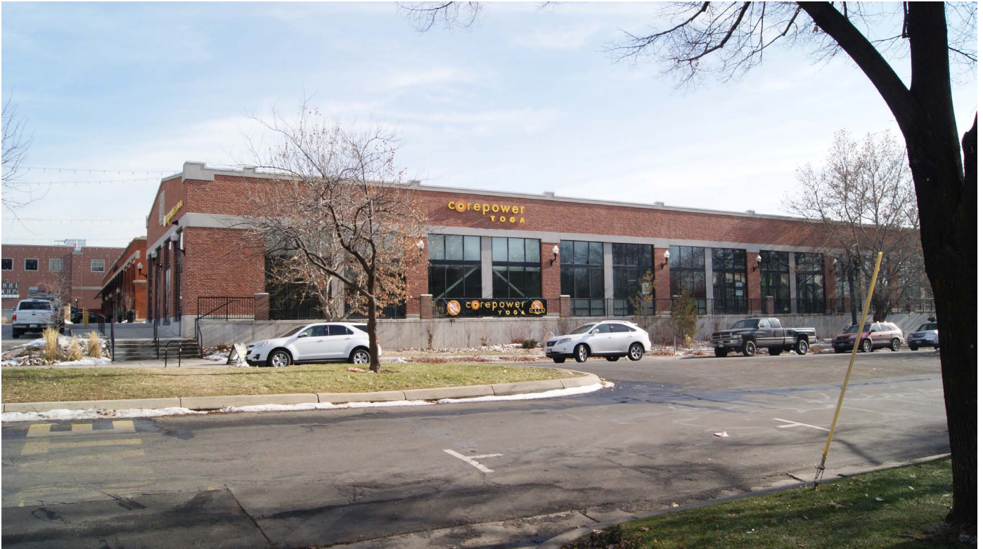
West elevation view from 600 east. The subject property has space for up to 5 tenants.
