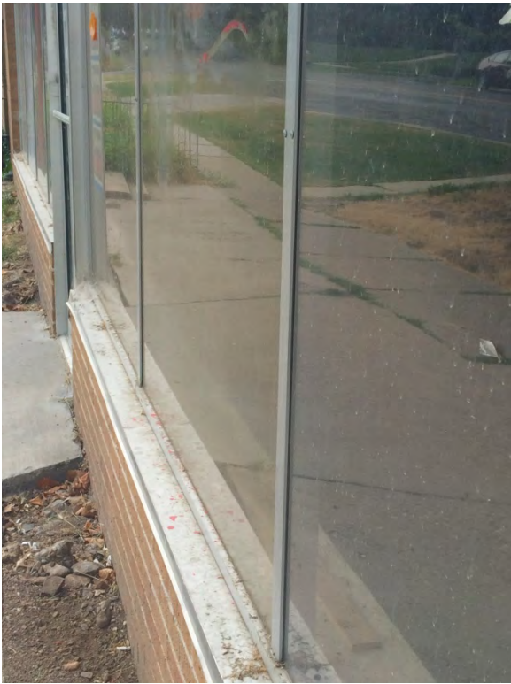
Close-up view of existing aluminum framed storefront windows
