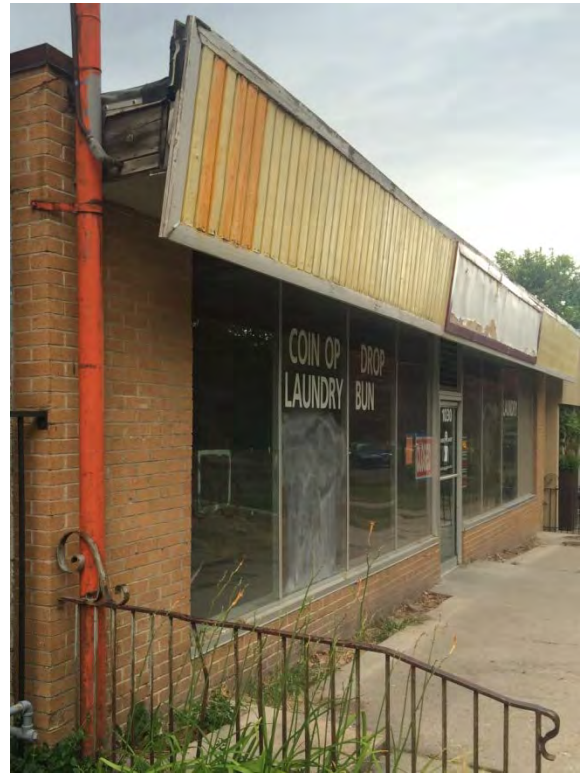
View of existing wood fascia
