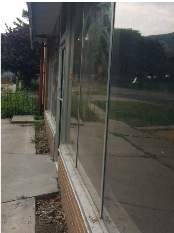
Existing building profile looking east
