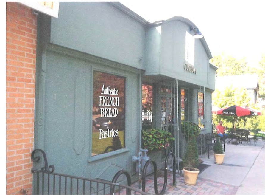
EXISTING DELI FACADE
