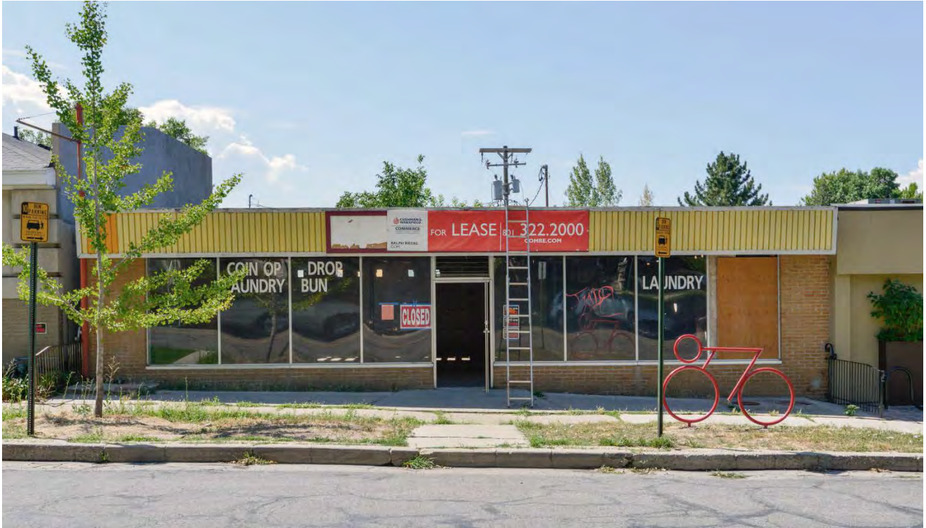
Existing facade of the subject property
