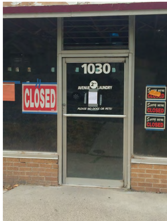
Existing single aluminum framed glass door
