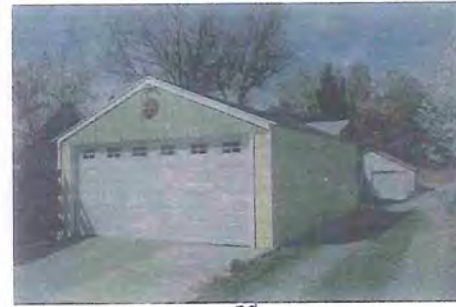
1037 E 2 nd Avenue (garage)
