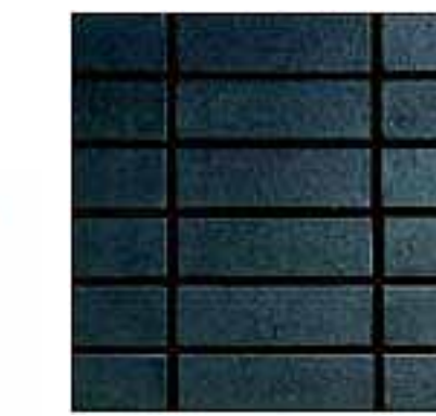
Stack Bond glazed brick on street elevation.
