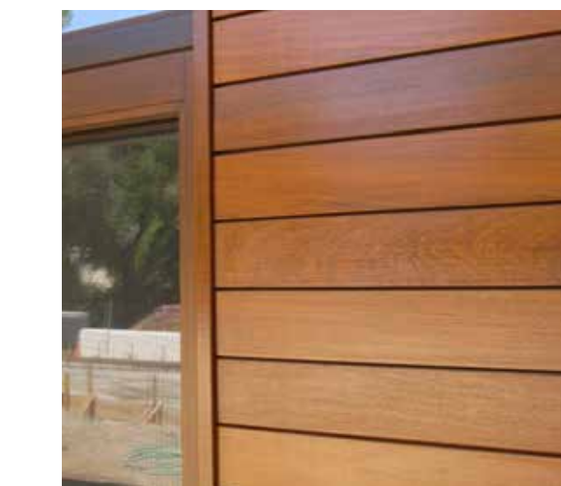
Horizontal wood rainscreen siding, stained finish.
