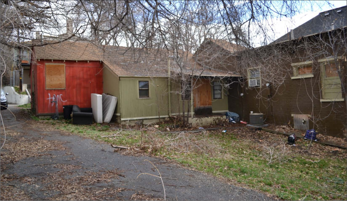
APPLICATION SITE & EXISTING STRUCTURE - FROM THE REAR
