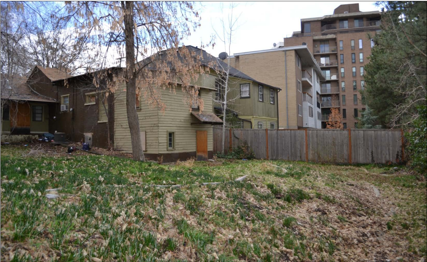
EXISTING SITE & STRUCTURE - FROM THE REAR LOOKING SOUTH EAST
