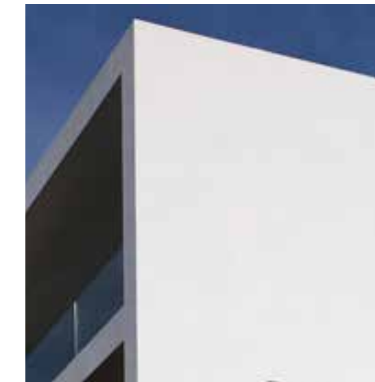
Smooth white stucco with acrylic top coat at soffits, wall returns, garage and master bedroom.
