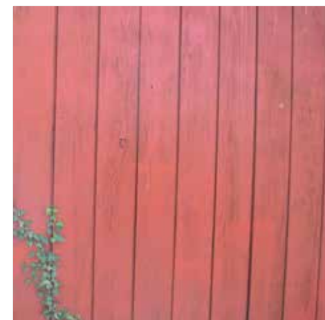
Red vertical wood siding over brick or framing
