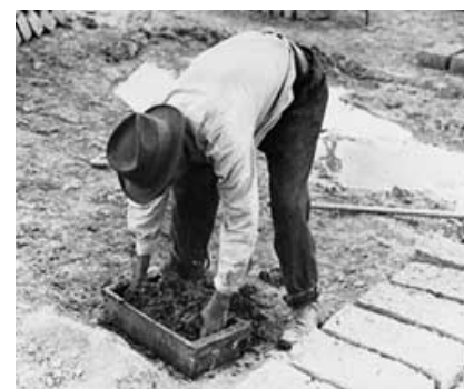
A mixture of mud and straw is pressed into a mold to form an adobe brick. After the adobe brick is removed from the mold, it must dry in the open air for a month or more before it can be used. Photo: Russell Lee, Farm Security Administration Collection, Library of Congress.
