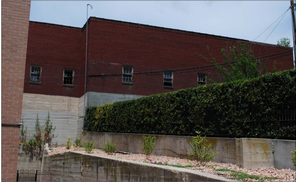
SOUTH FAÇADE OF PARKING GARAGE
