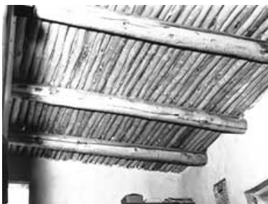
Viga logs and savinos are seen in the interior of the adobe building. Often the wooden materials that comprise the traditional flat adobe roof create interesting and pleasing patterns on the ceilings of interior rooms. Photo: Russell Lee, Farm Security Administration Collection, Library of Congress
