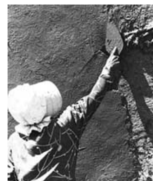
Traditional adobe repair. Photo: Russell Lee, Farm Security Administration Collection, Library of Congress.
