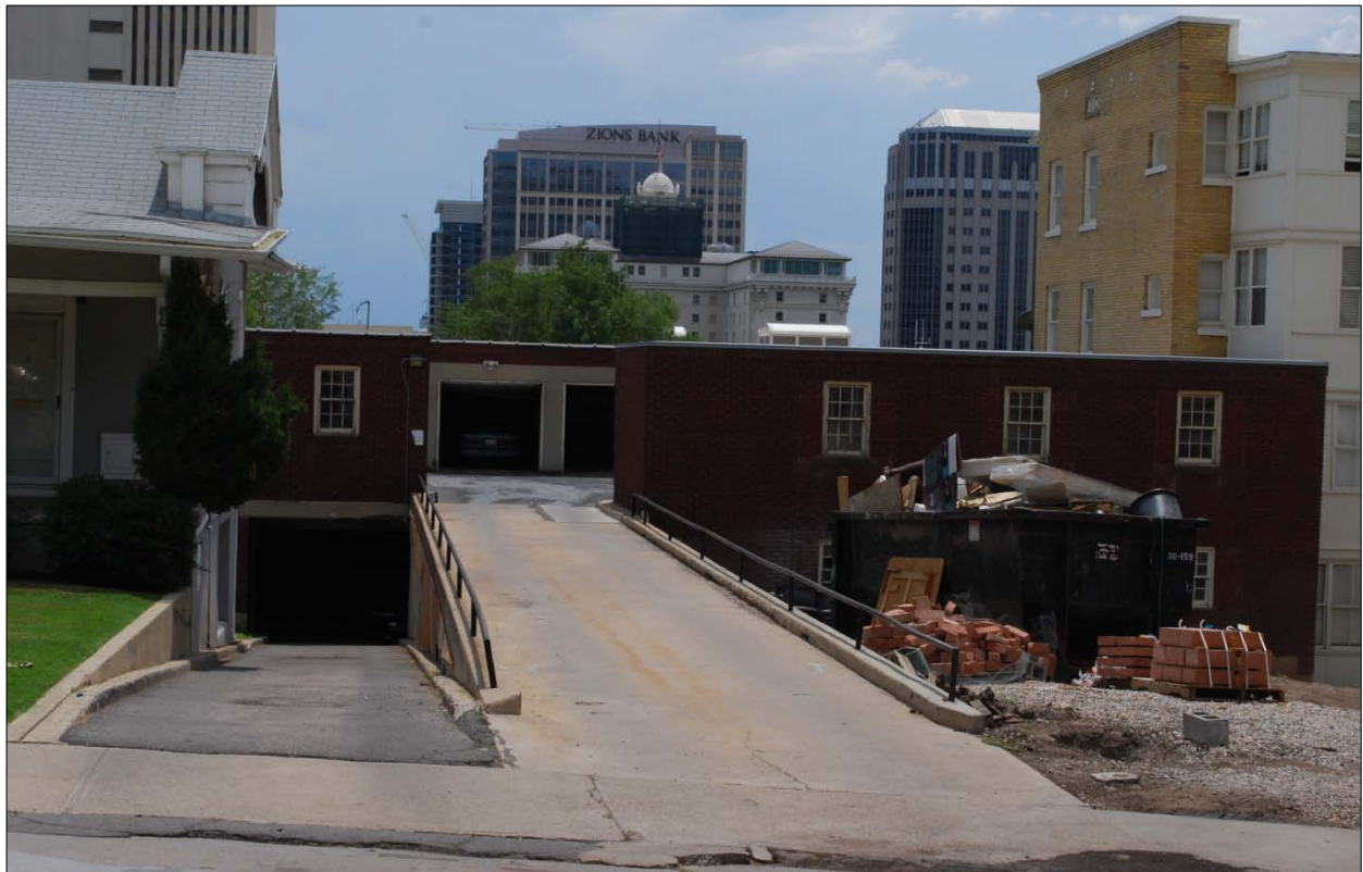
KENSINGTON APARTMENTS PARKING GARAGE FROM 200 NORTH
