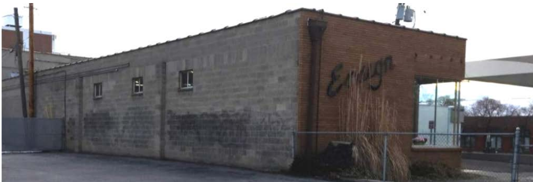
Existing North Façade
