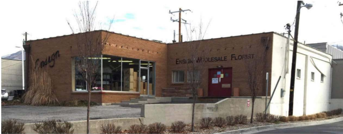
Existing West Façade
