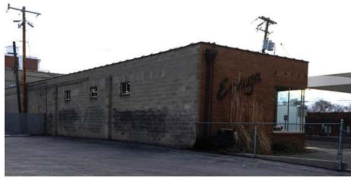
EXISTING NORTH FACADE
