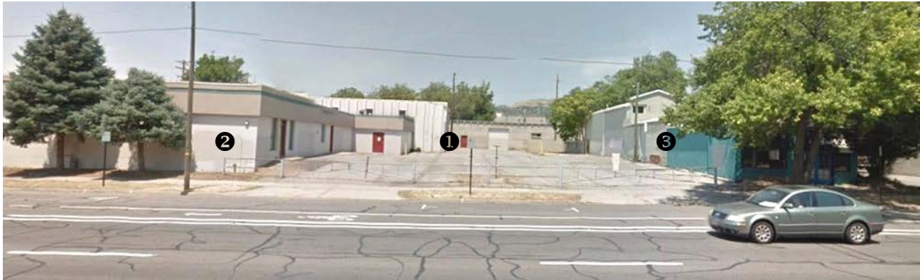
Existing Buildings to be Demolished
