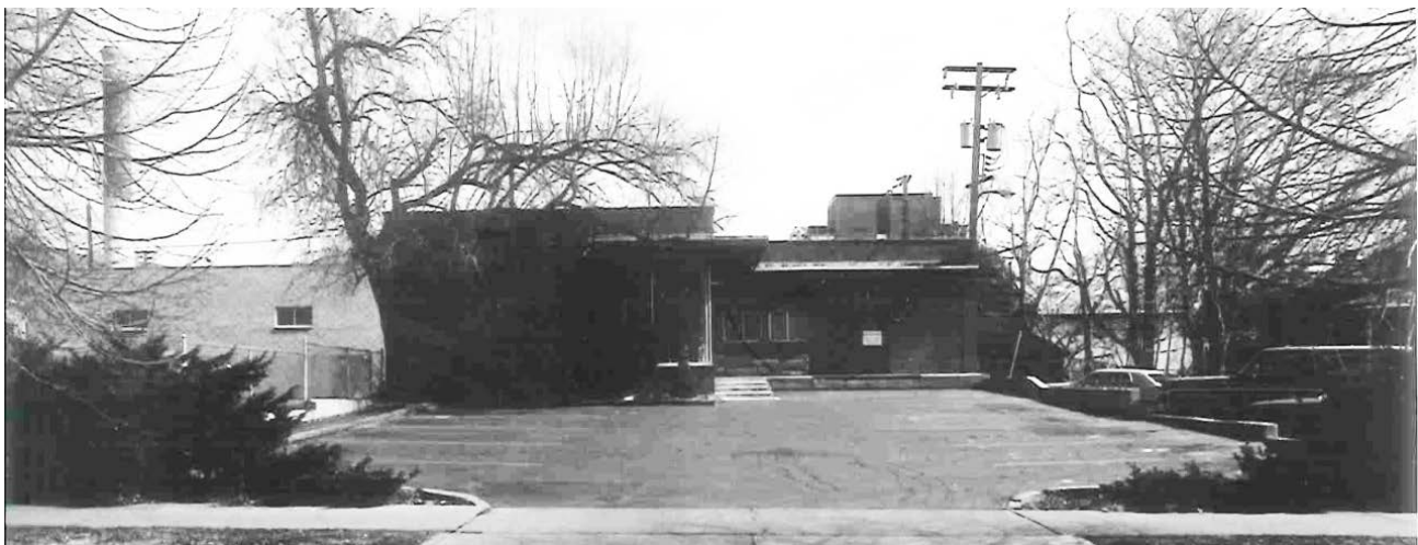
Photo of Existing Building with Canopy
