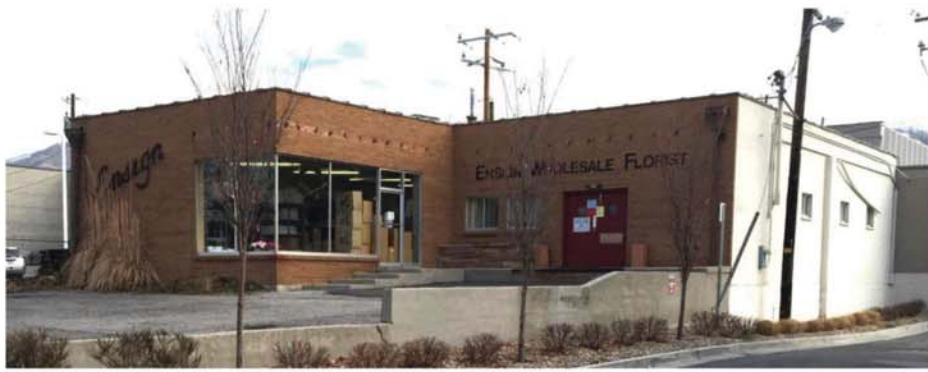
EXISTING WEST FACADE
