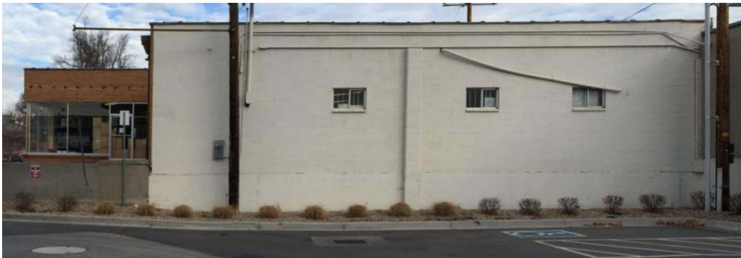
Existing South Façade
