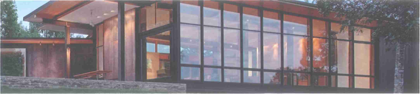
ABOVE // CARLTON ARCHITECTURE, NC
