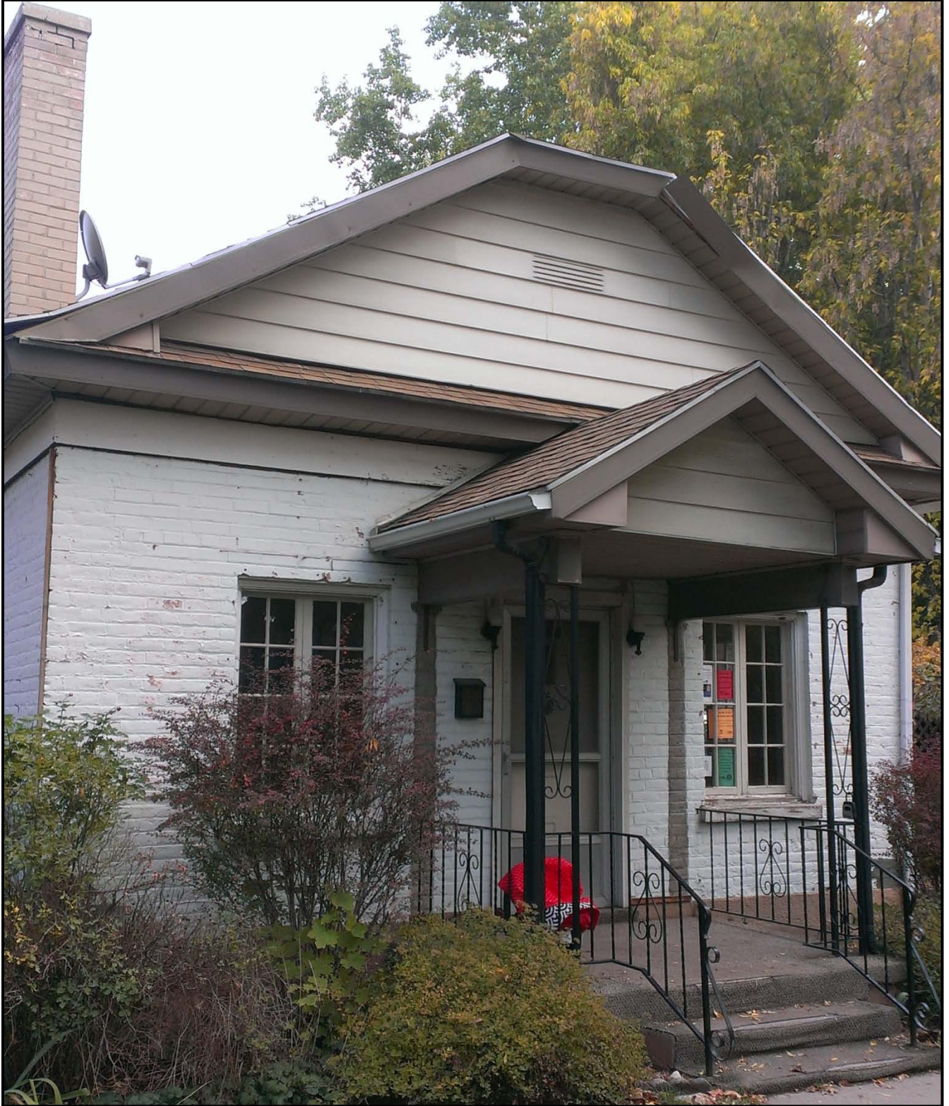
RECENT - ALUMINUM CLADDING REMOVED
