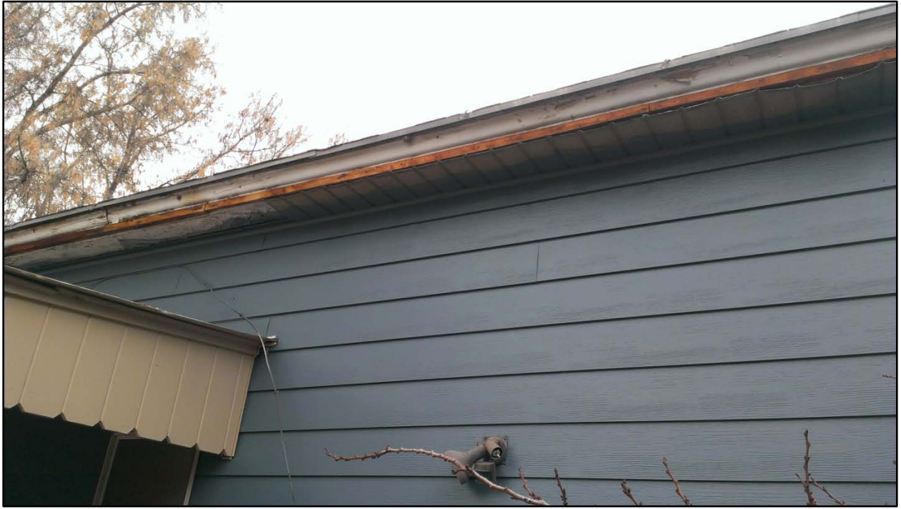
CURRENT - REAR FAÇADE
