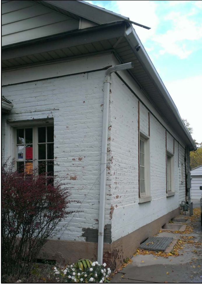
RECENT - ALUMINUM CLADDING REMOVED
