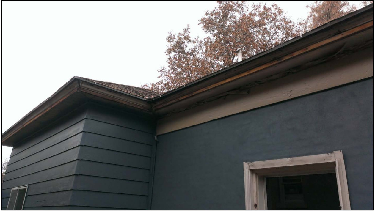
CURRENT - NORTH FAÇADE
