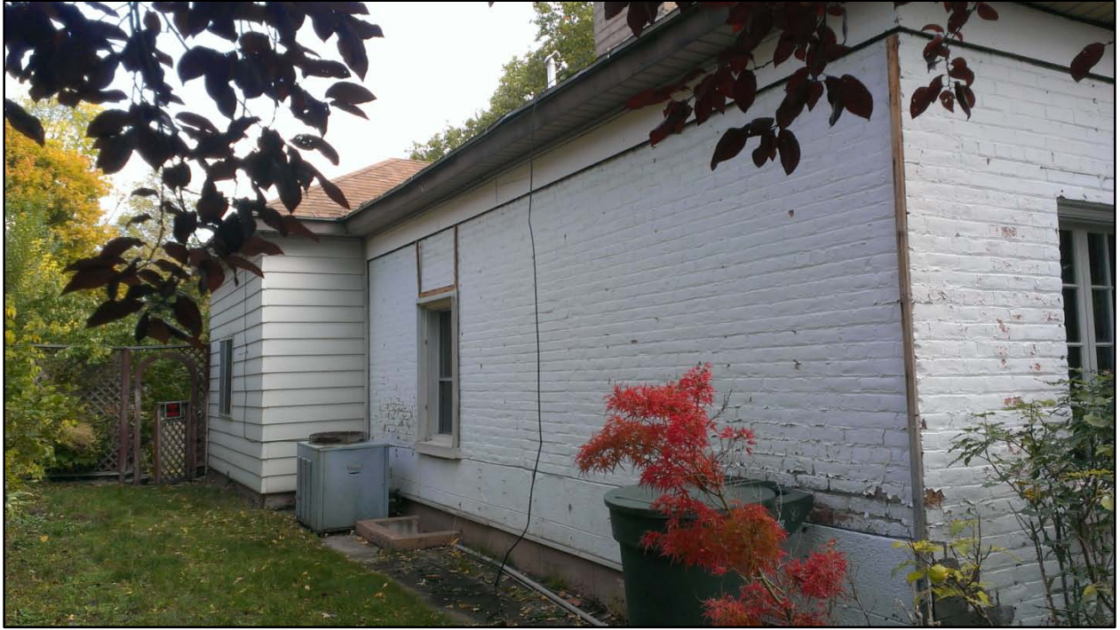
RECENT - ALUMINUM CLADDING REMOVED
