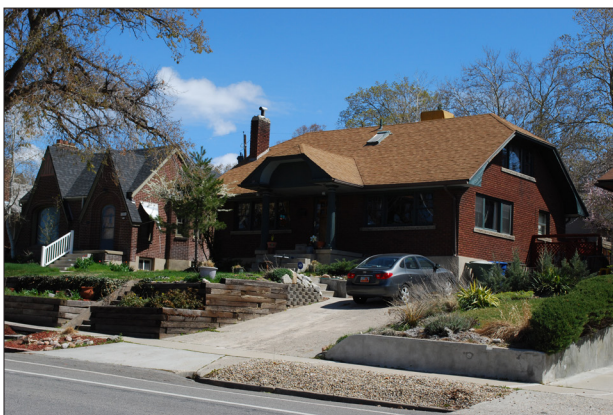
The second development phase provides contrasting period revival designs and often an increase in building height.
