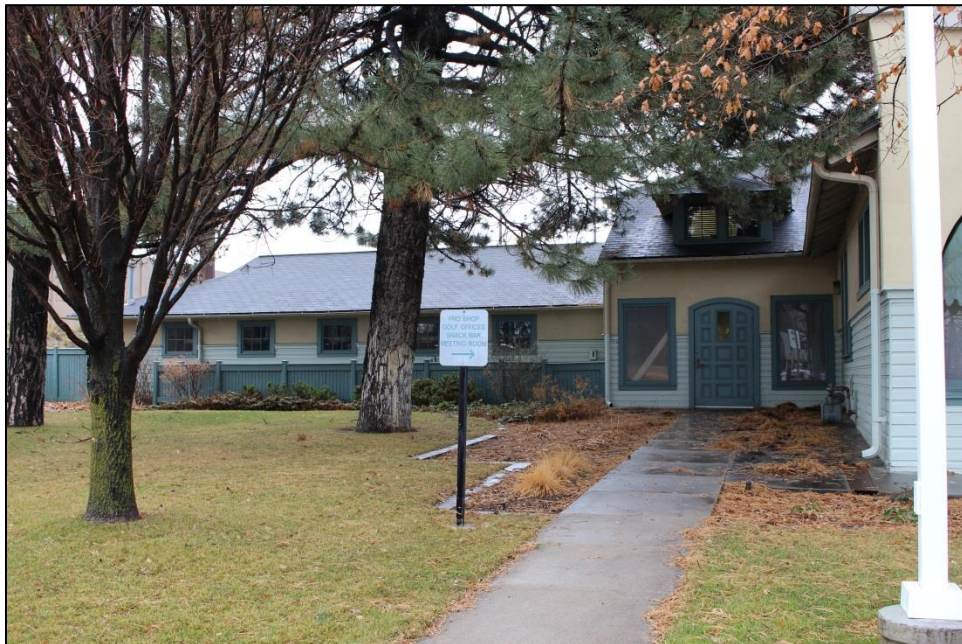
Photograph 10. West elevation of clubhouse northern ell and garage addition (2015); looking east
