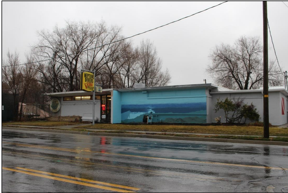
Photograph 22. Non-contributing commercial building—Building 2 (2015); looking northeast
