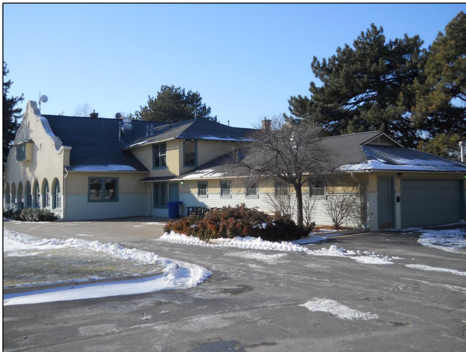
Photograph 8. Overview of clubhouse (2015); looking southwest
