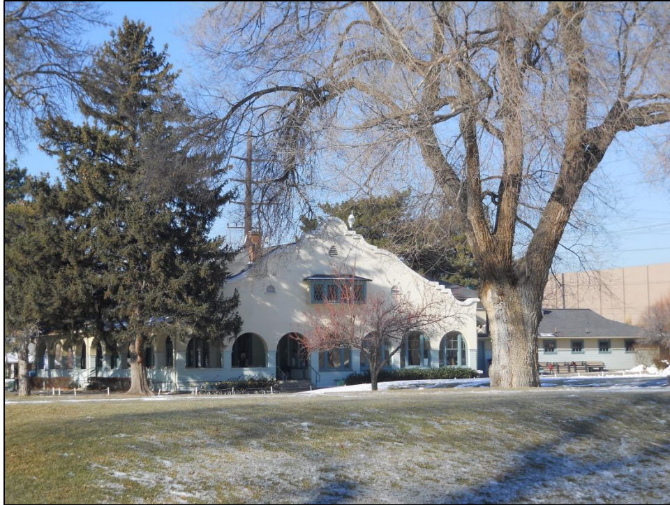
Photograph 7. Overview of clubhouse (2015); looking northwest
