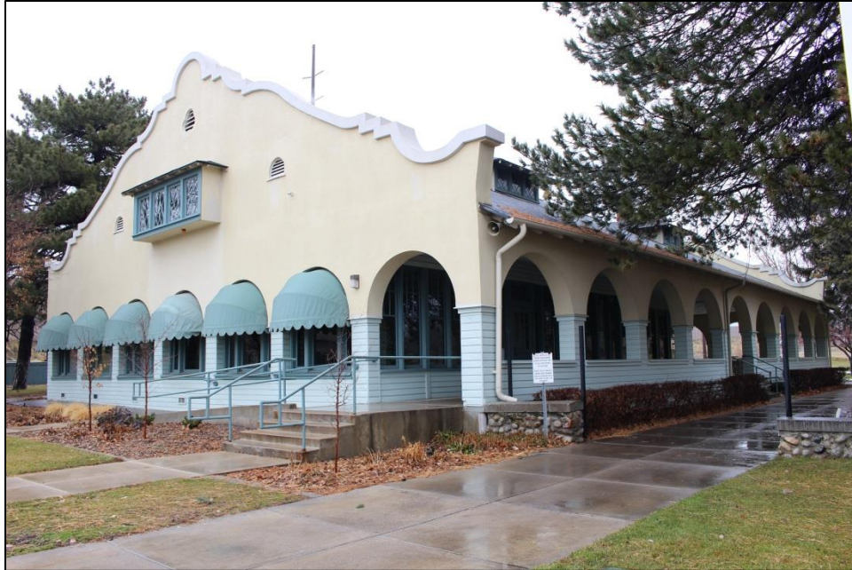
Photograph 17. West and south elevations of clubhouse (2015); note veranda along south elevation; looking northeast
