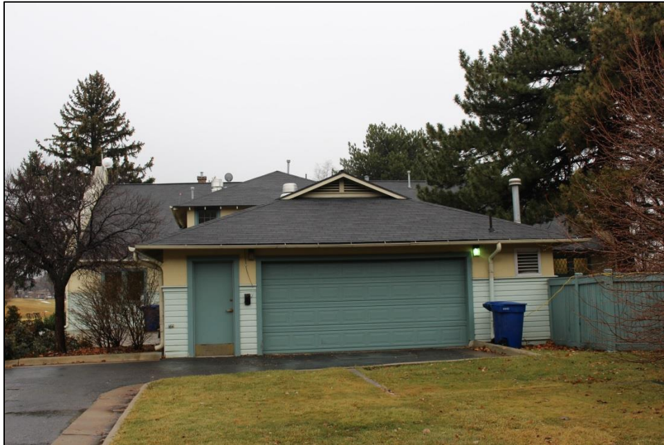
Photograph 15. North elevation of clubhouse with garage addition in foreground (2015); looking south
