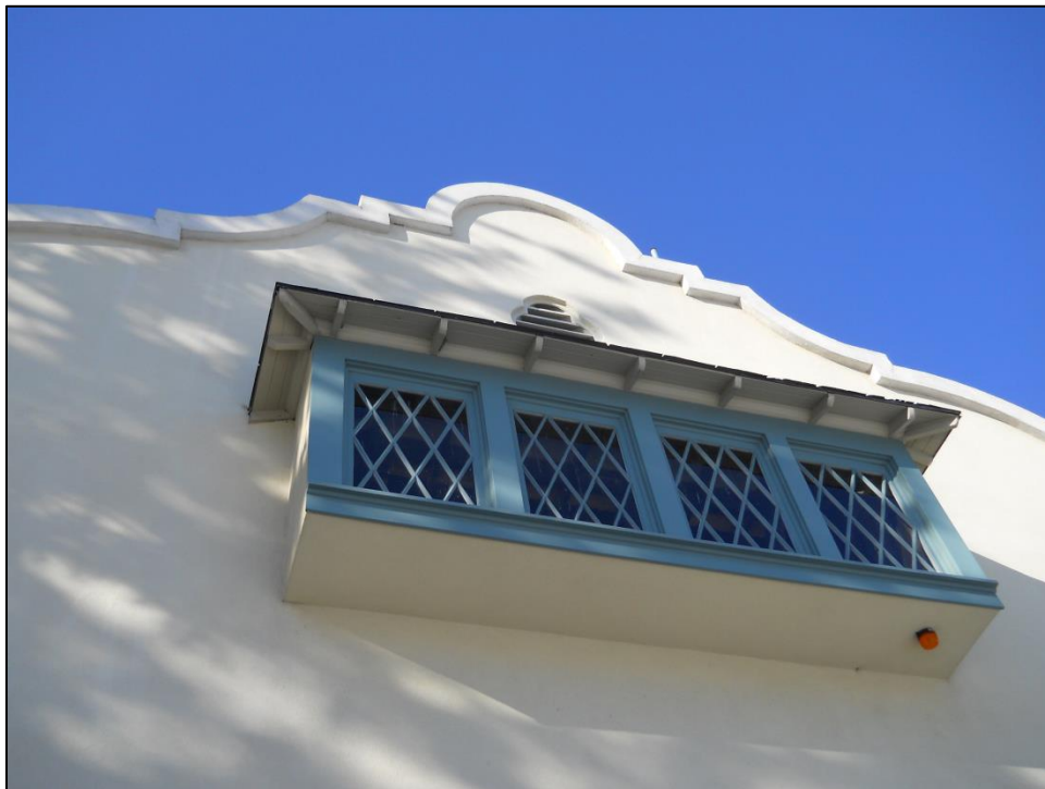
Photograph 16. Example of window detail on east elevation of clubhouse (2015); looking west
