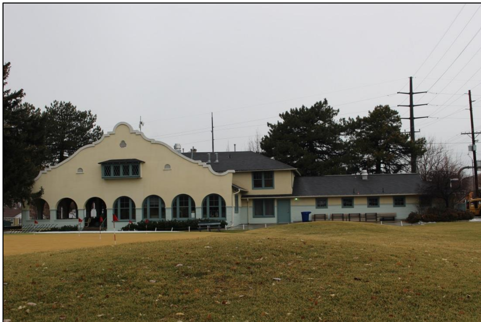
Photograph 12. East elevation of clubhouse (2015); looking west
