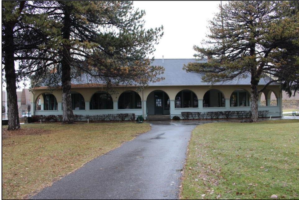
Photograph 11. South elevation of clubhouse (2015); looking north
