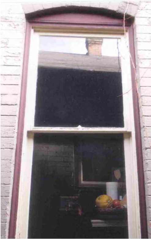
West Elevation Window to be replaced
