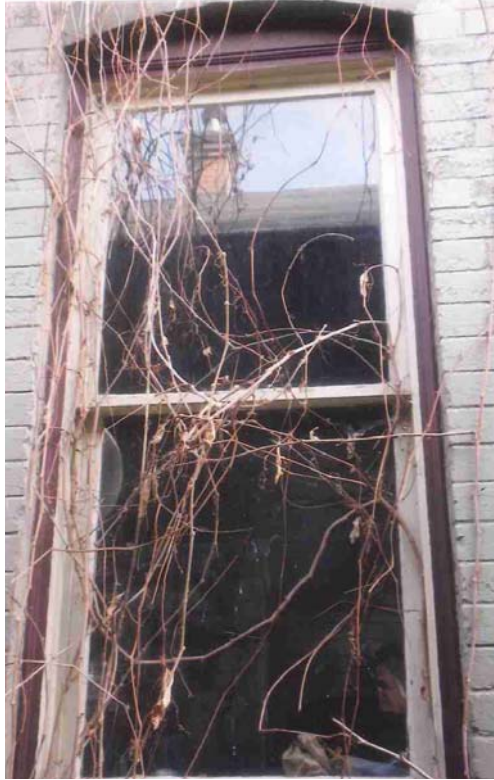
West Elevation Window to be bricked-in
