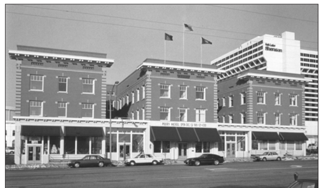
Peery Hotel, c. 1910, Charles Onderdonck, architect, Salt Lake City, Salt Lake County. This example of the “E” or Double Court was built for Ogden Businessmen David and Joseph Peery.
