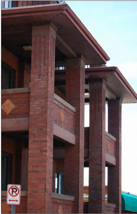
Well defined and detailed projecting balconies help to establish building form and scale.
