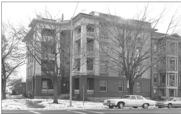
Apartment building, C. 1910, Salt Lake City, Salt Lake County. Another example of the "L" configuration, this block has a small forecourt at the corner of the lot. The projecting porches are supported, starting at the second floor, with tapered square Ionic columns that frame the corner entry.
