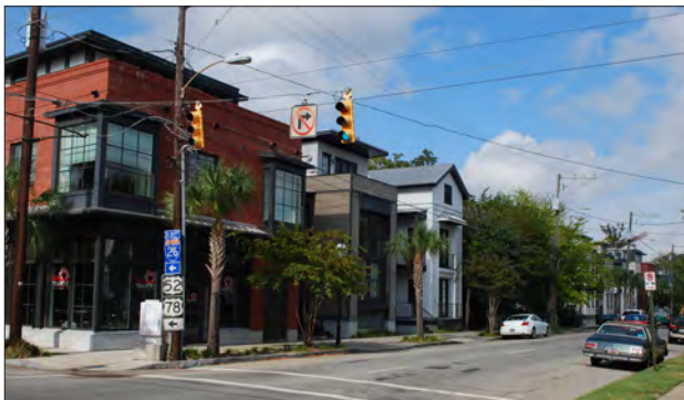
A horizontal corner emphasis frames a series of vertically proportioned street facades.
