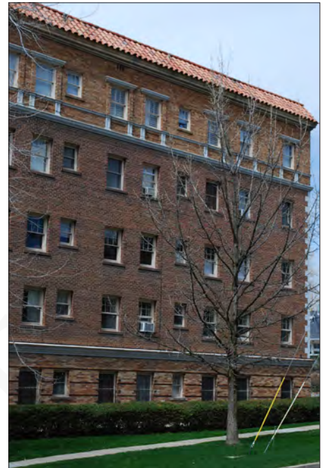
Differentiation in the design of the first floor and the top floor with tiled roof parapet help to frame the façade and reduce the perception of height.
