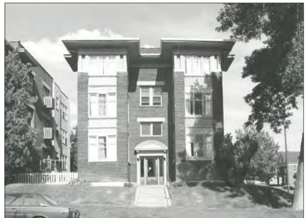
Norma Deane Apartments, 1917, Salt Lake City, Salt Lake County. One of three identical buildings on the same site built for the State Loan and Trust by C. C. Severs, this block exhibits the wide overhanging eave and geometric woodwork common to the Prairie School Style.
