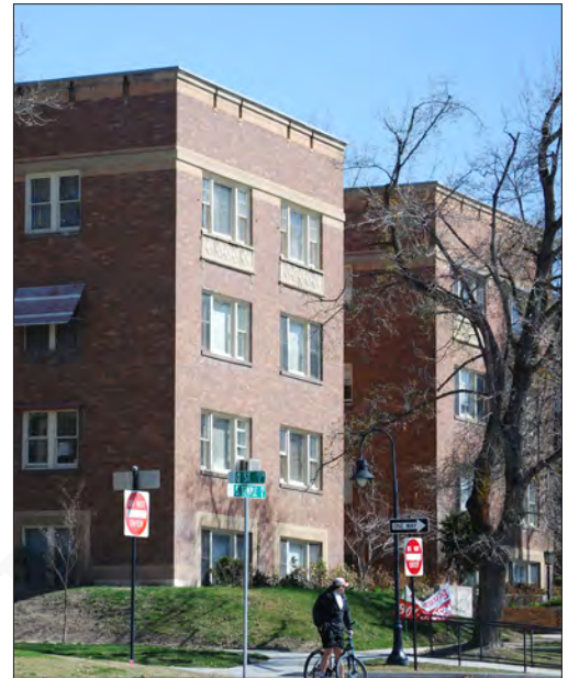
Symmetrical projecting wings of the primary street facade enclose a central recessed entrance court.
