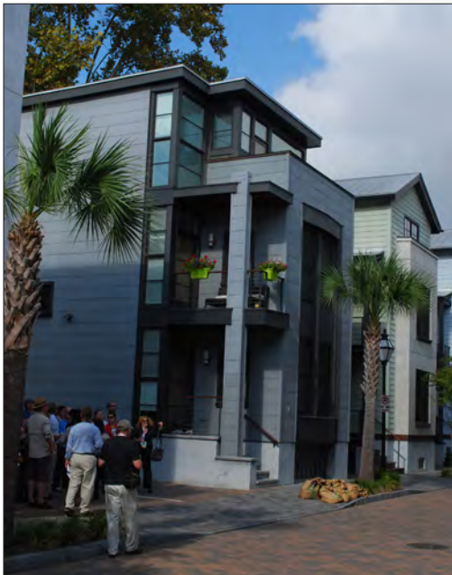
Porch and balcony are jointly defined here, and introduce outdoor terrace space above.
