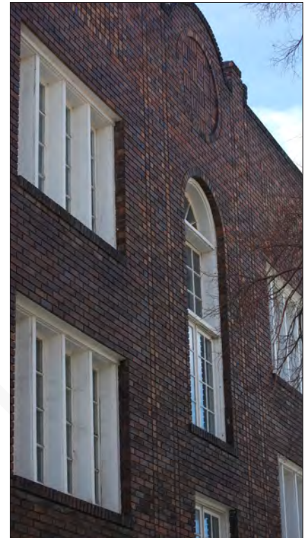
Stone window reveals and mullion subdivision contrast with the dark brickwork of the facade wall.
