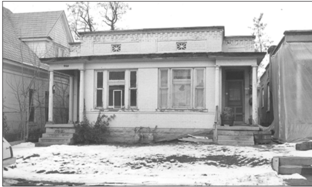
Double house, c. 1905, Salt Lake City, Salt Lake County. This single-story example of the double house has side entries with narrow porches supported by Tuscan columns.
