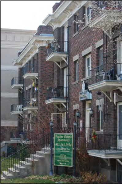
Symmetrical massing and composition, balconies and fenestration pattern combine to integrate with the street.
