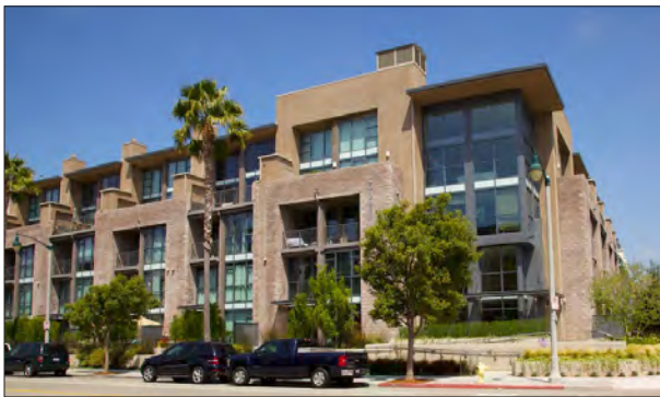
Stepping back the top floor combines with facade articulation and corner design focus to reduce perceived height and scale.
