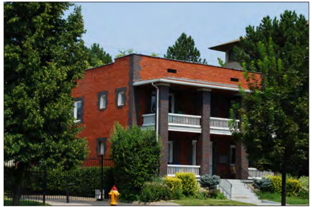
Contrasting materials and colors help to frame the building and the balcony portico while enhancing the contribution to the character of the street.
