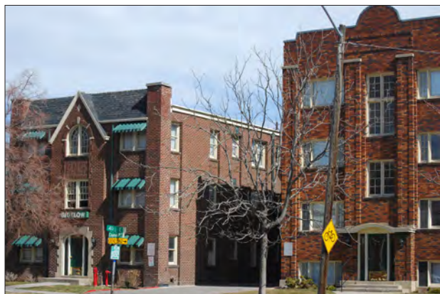
Despite contrasts in height and architectural style, the solid to void ratio and window scale and proportions help to establish a visual affinity and compatibility between the two buildings.
