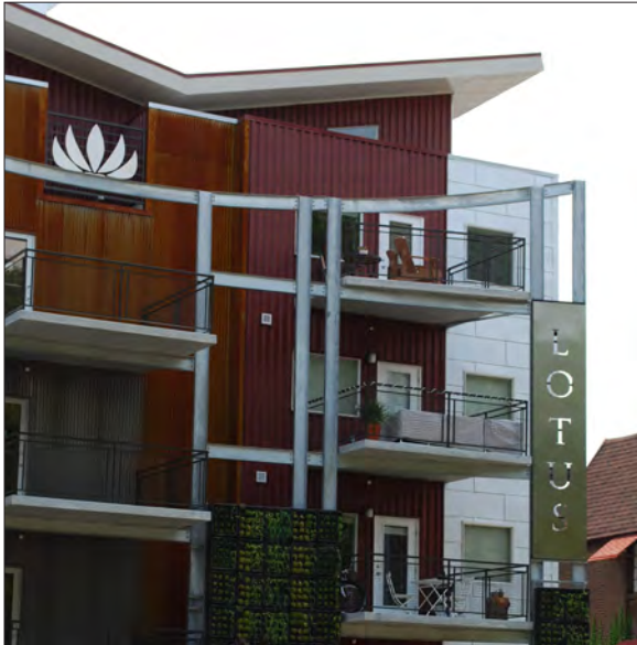
Sign lettering and motif are both used here as decorative detail to embellish the facade.
