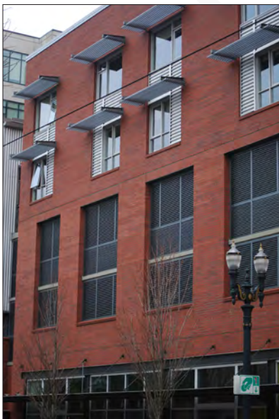
Utility equipment and areas can be discreetly planned and designed.
