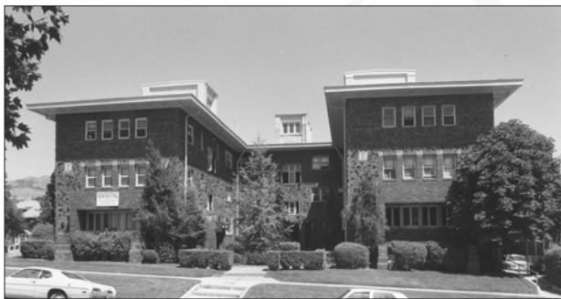
Caithness Apartments, 1908, Ware and Treganza, Architects, Salt Lake City, Salt Lake County. A “U” court design influenced by the Arts and Crafts and Prairie School styles, it originally featured an extensive roof garden.
