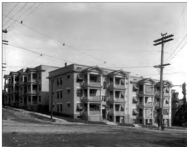
The Kensington Apartments were constructed about 1905, and represent a type of apartment known as a “walk-up.”
