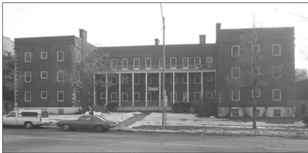
Bell Wines Apartments, 1927, Slack Winburn, architect, Salt Lake City, Salt Lake County. This “H”-type apartment block is preceded by an unusually shallow forecourt. A tall portico supported by square columns spans the width of the court. The wings of the building are emphasized by stone quoins and a molded cornice.
